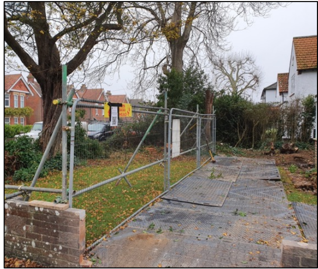
GP2: Tree protection barriers & trackmat ground protection
