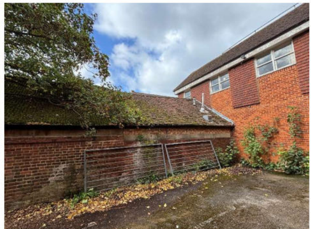
Image 3 – View of north-east elevation
