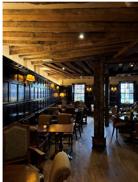
Figure 8 and 9: The site of the former alley way between the 15 th Century timber framed buildings. Internal view of the timber framing of the south-western building.
