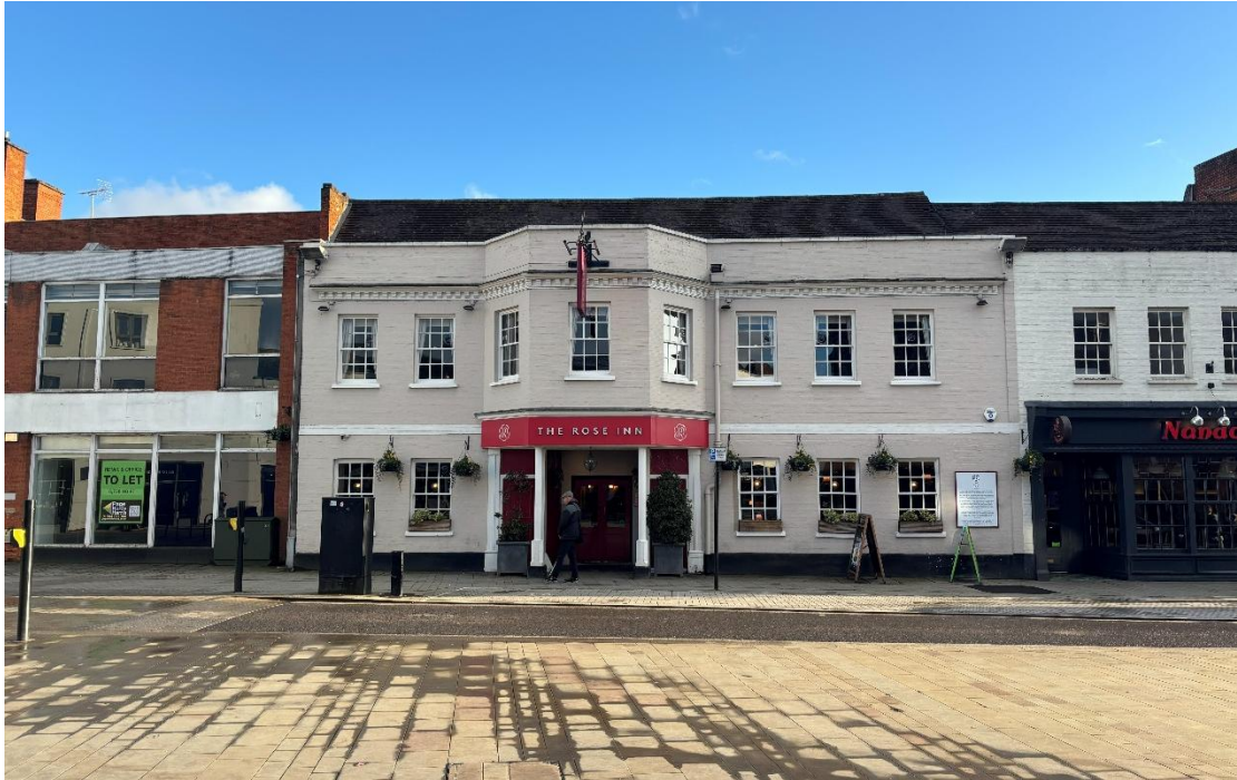
Figure 7: Front elevation of The Rose, the entrance demarking the medieval alley between the two former buildings
