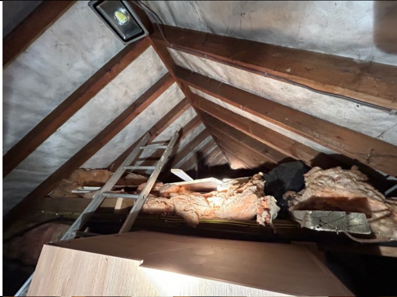
Photograph 4: Loft void within the bungalow showing the wooden supports and the Tyvec lining.
