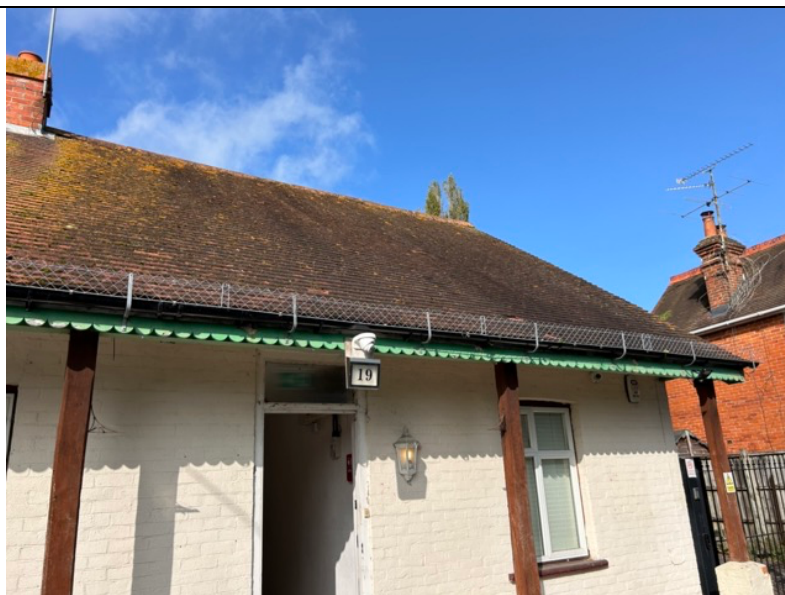
Photograph 1: Front / east side of the bungalow.
