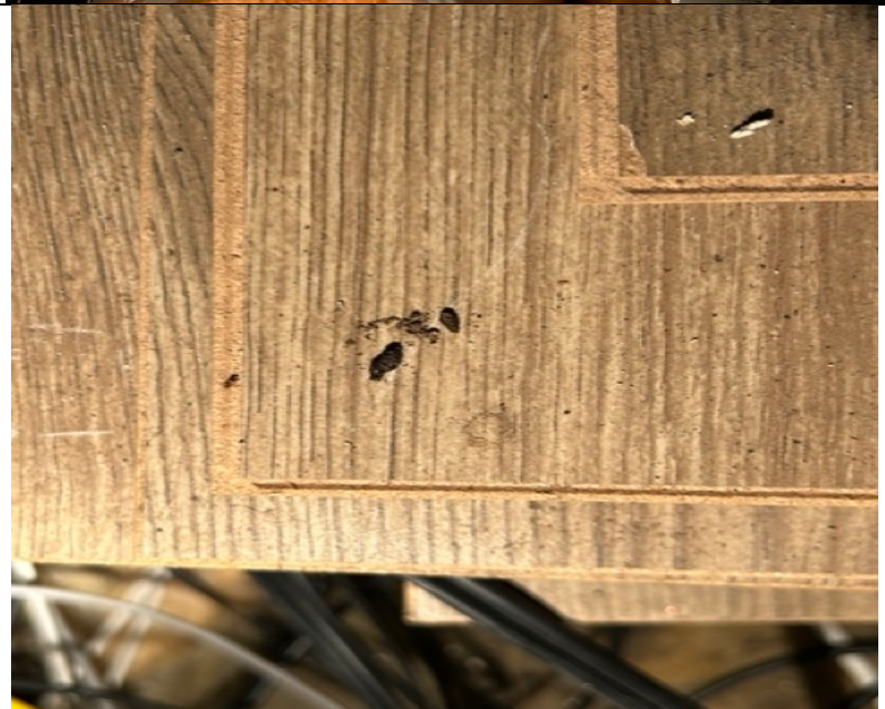
Photograph 6: Bat droppings found within the loft void.
