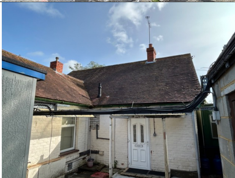
Photograph 3: Back / west facing side of the bungalow.
