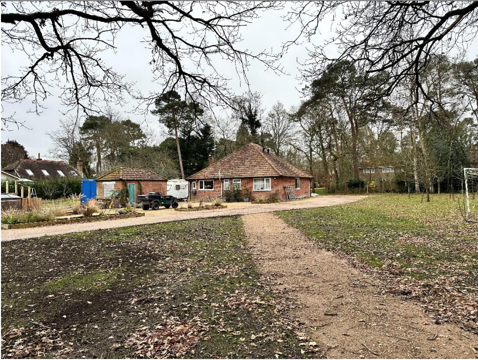
Overview of the house from the location of T7
