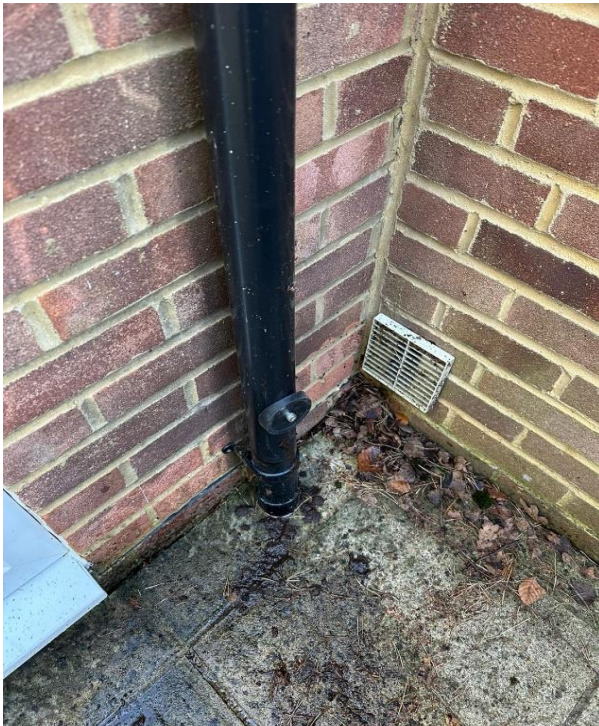
RWP2 access cut
