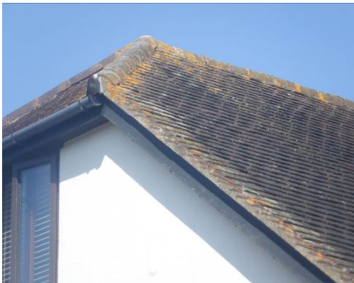
Photograph 7. Merge mortar intact at the verges to the rear of the property
