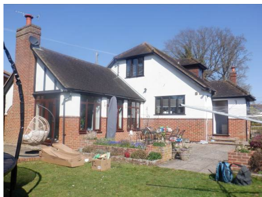
Photograph 2. Rear of property viewed from the south.
