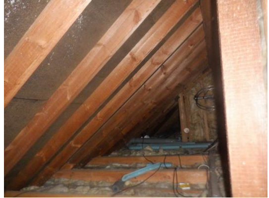
Photograph 14. Fiberglass insulation on the floor and walls
