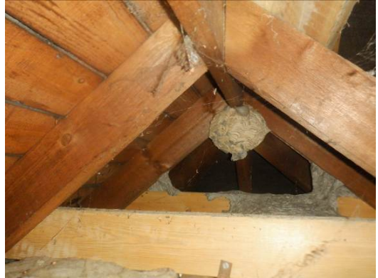
Photograph 13. Roof void with fibreglass insulation covering the floor
