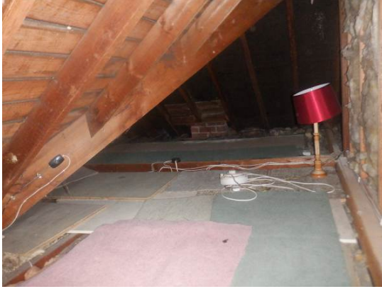
Photograph 13. Carpeted entrance in eaves space
