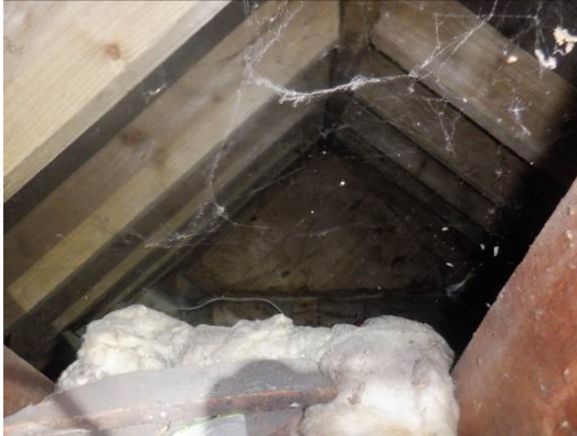
Photograph 15. Central gable lined with timber cladding with small amounts of visible daylight
