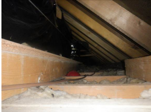
Photograph 12. Roof void with fibreglass insulation covering the floor
