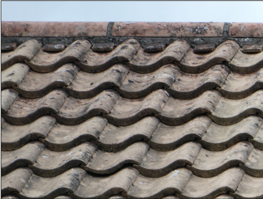
Figure 5. Example of ridge tiles. Frankforte, Three Mile Cross. 11.07.23
