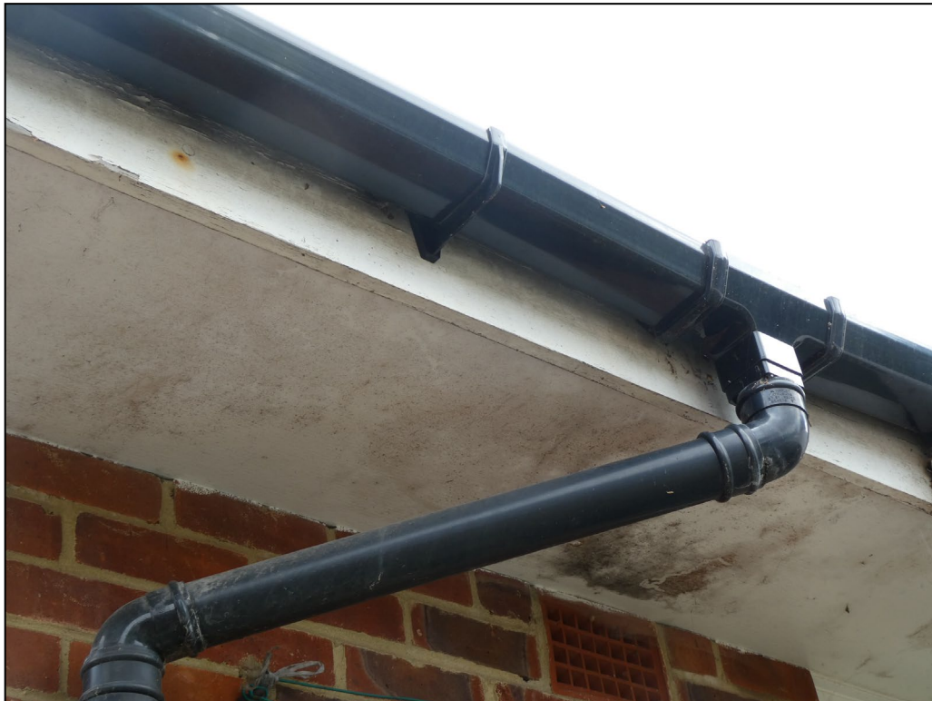
Figure 8. Soffits and fascias. Frankforte, Three Mile Cross. 11.07.23
