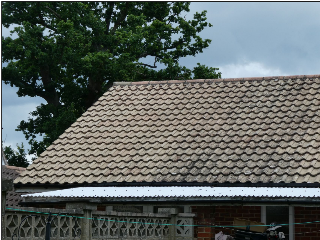
Figure 4. Example of roof tiles. Frankforte, Three Mile Cross. 11.07.23
