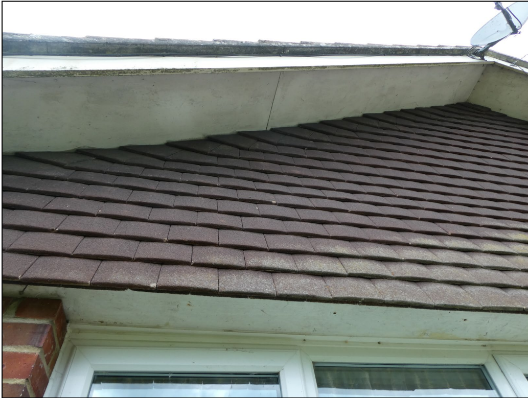
Figure 7. Example well fitted hanging tiles. Frankforte, Three Mile Cross. 11.07.23
