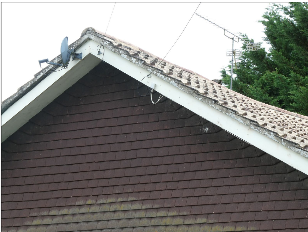
Figure 6. Example of verges. Frankforte, Three Mile Cross. 11.07.23
