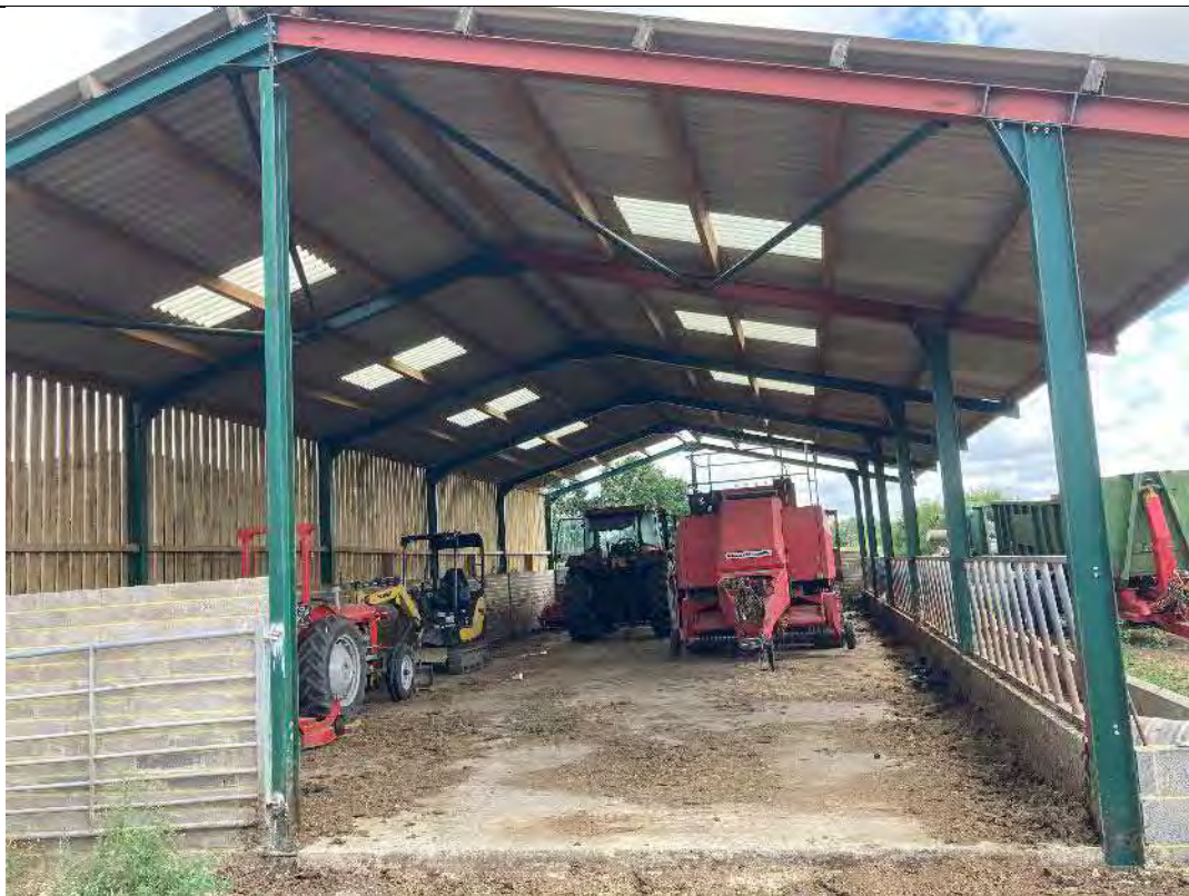
Photograph 10 – Barn 3 used for vehicle storage (facing south)
