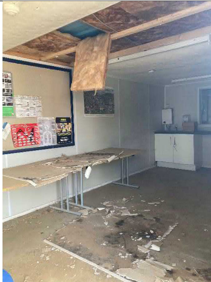
Photograph 19 – Internal area of the open metal container within Area 2
