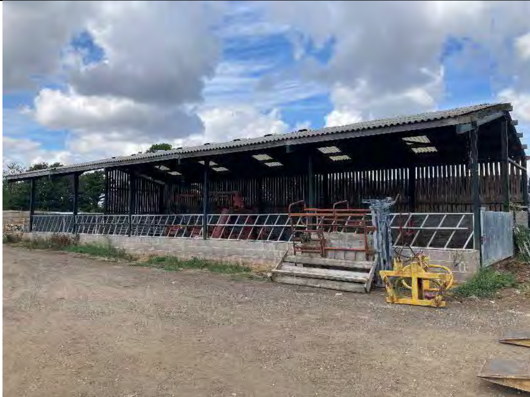
Photograph 9 – External view of Barn 2 (facing southwest)
