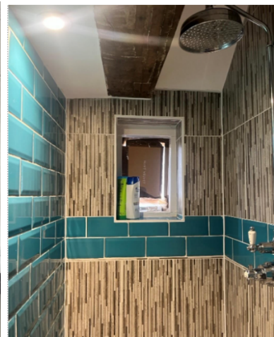
2 nd floor shower room (not WC room)
