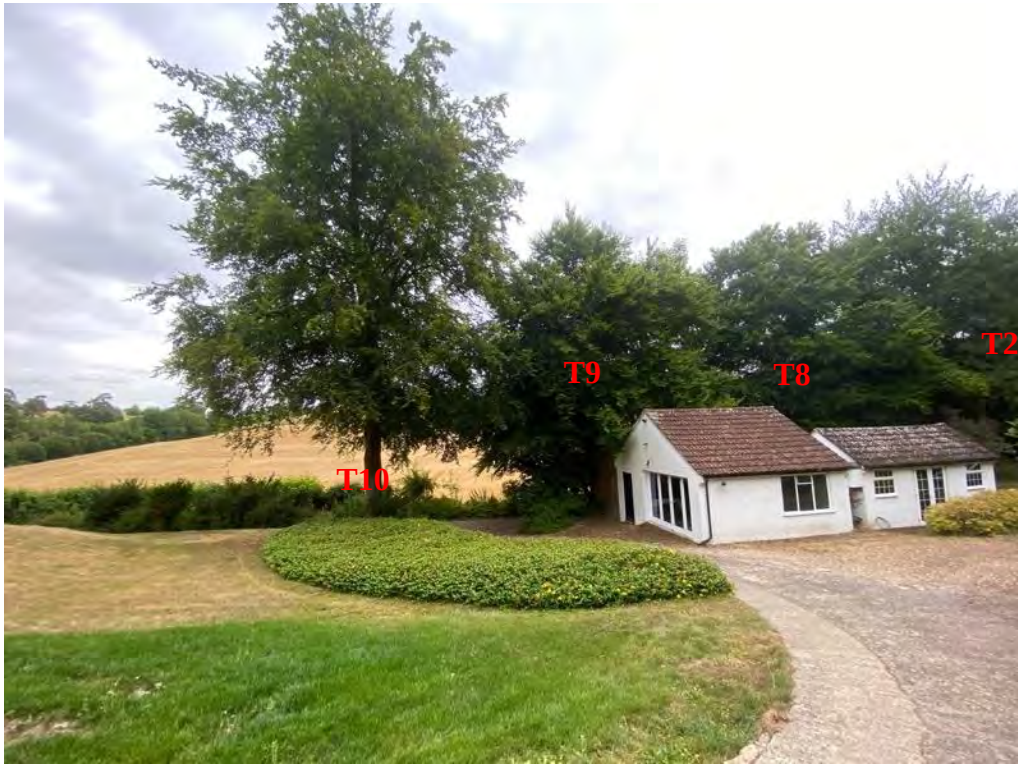
Photoview 15: View east at existing drive and annex building.
