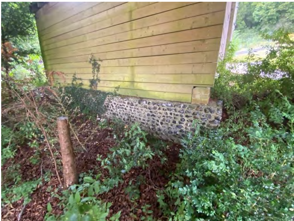
Photoview 14: View west at existing annex structure near T8 and T9.
