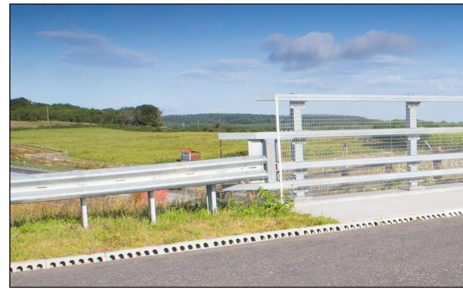
DETAIL 1 - PARAPET TO SAFETY BARRIER TRANSITION
