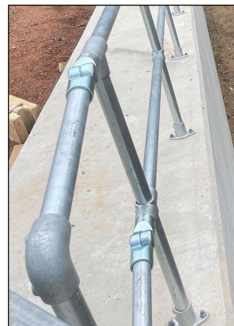
DETAIL 9 - GUARD RAIL ON WINGWALLS (SEE NOTE 4)
