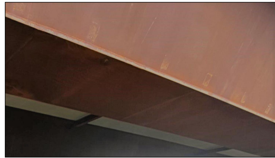
DETAIL 3 - WEATHERING STEEL BOX GIRDER (SEE NOTE 4)
