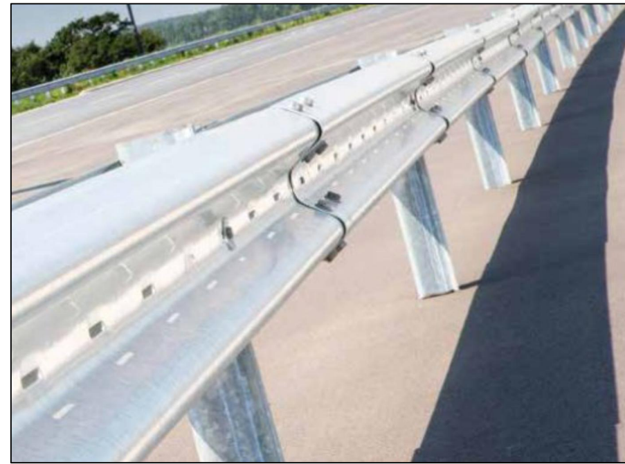
DETAIL 2 - SAFETY BARRIER
