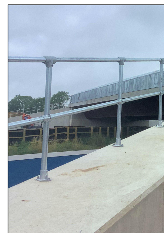
DETAIL 10 - GUARD RAIL ON WINGWALLS (SEE NOTE 4)
