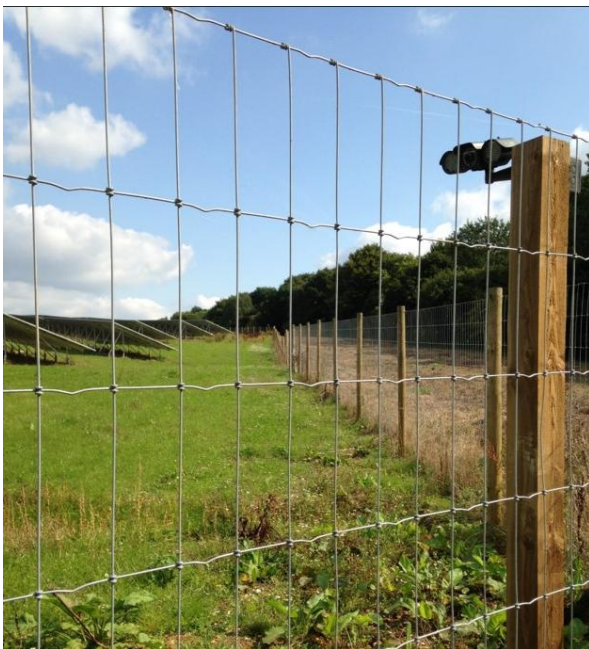
Plate 1: Example of timber fence posts with galvanised steel wire mesh fencing.
