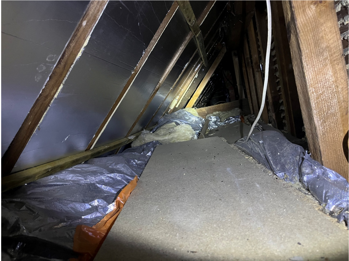
Figure 8. Interior of roof looking south
