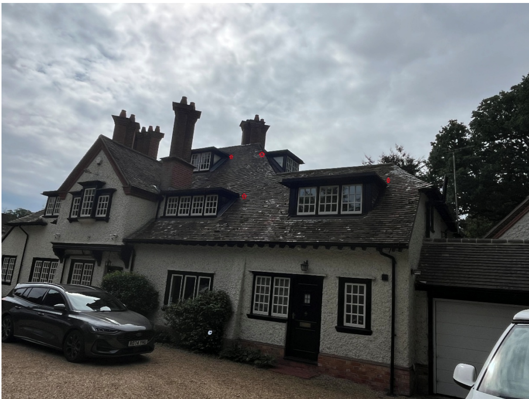
Figure 4. Western elevations looking east: Red arrows indicate potential openings for crevice roosting bats.
