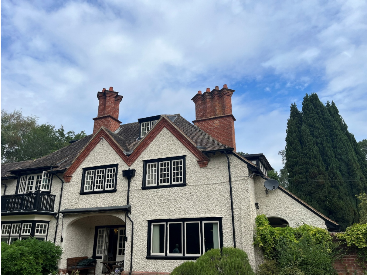
Figure 6. Detail of south valley looking southeast: Red arrows indicate potential openings for crevice roosting bats.
