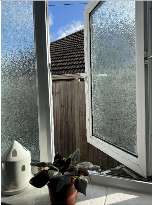
Open Downstairs Bathroom Window
