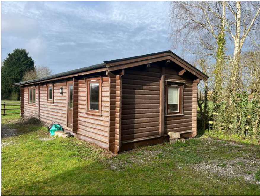
Photograph 2: Showing the mobile home log cabin to be removed.
