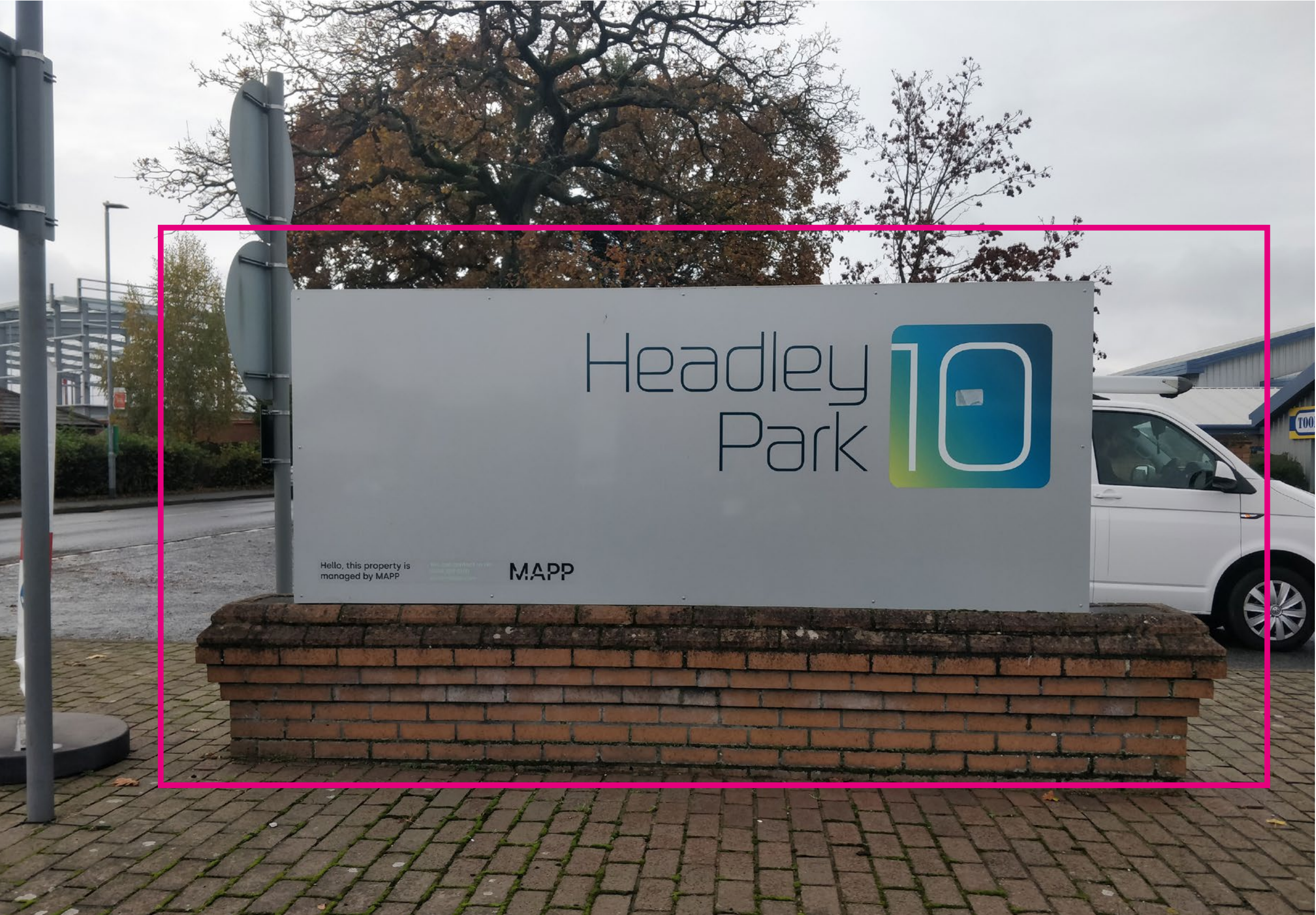
Signage to be removed and replaced.
