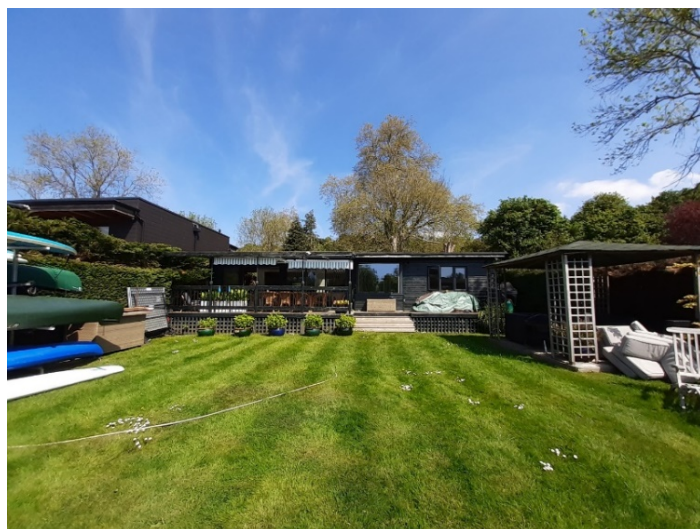
Figure 1 View of cabin and river from riverbank
