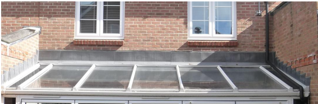
(Existing glazed panel roof)
