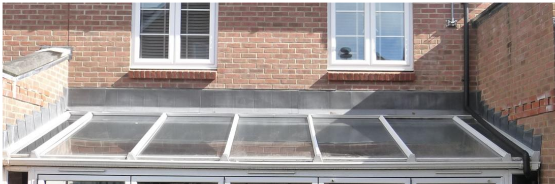
Existing Glazed panels and parapet walls.
