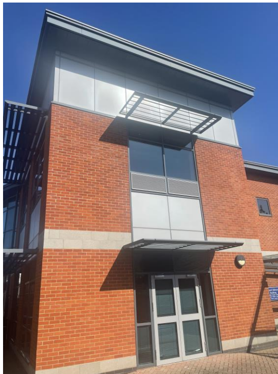
Existing Façade to adjacent Richard Aldworth Building – grey composite panels with brick walling
