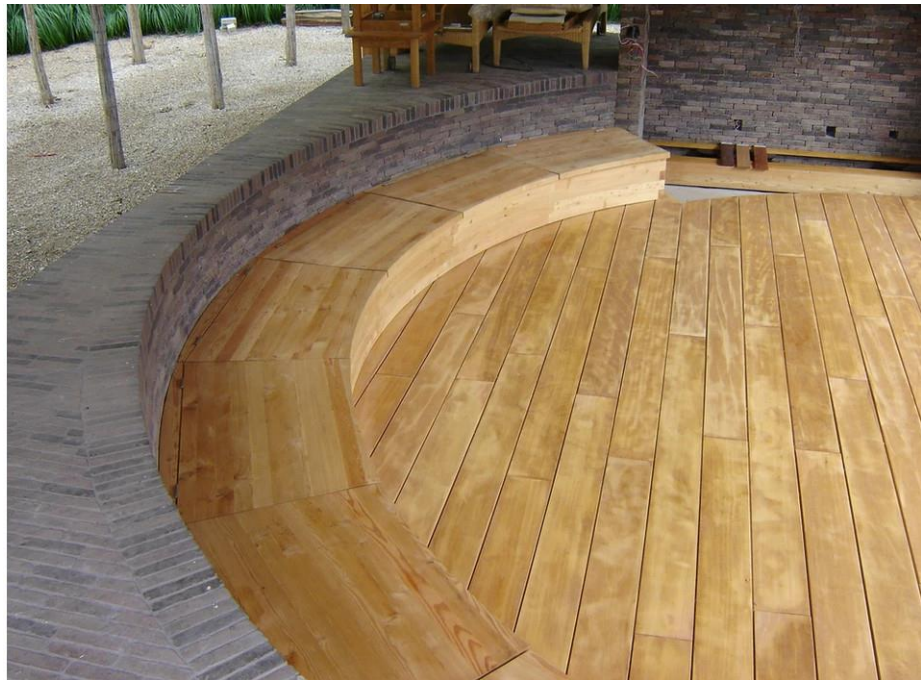
Example of built in seating areas to West Terrace
