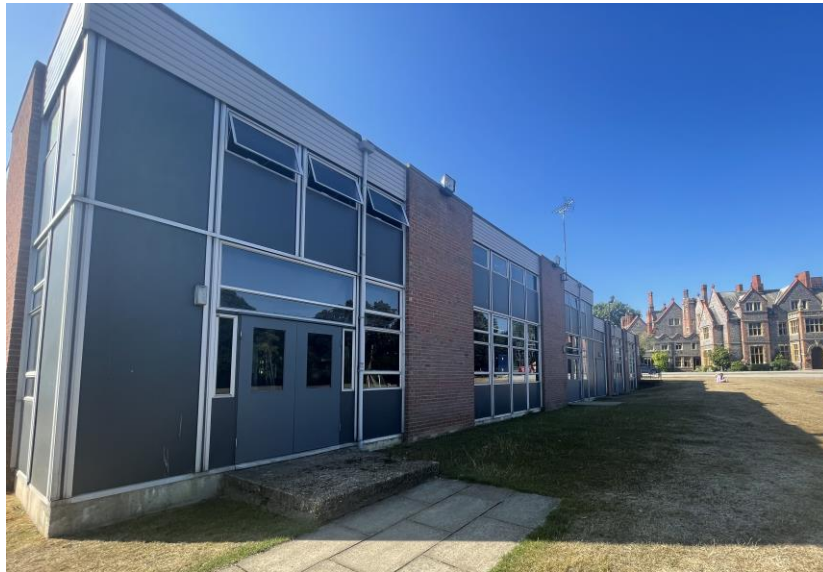
Existing Façade to Way Hall – grey composite panels with brick infill panels
