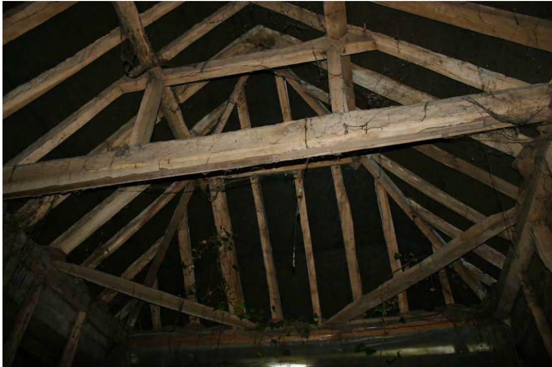
The roof of the midstrey. Looking NW.
