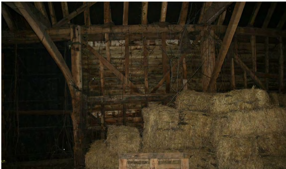
Wall frames in Bays 1 and 2, south side.
