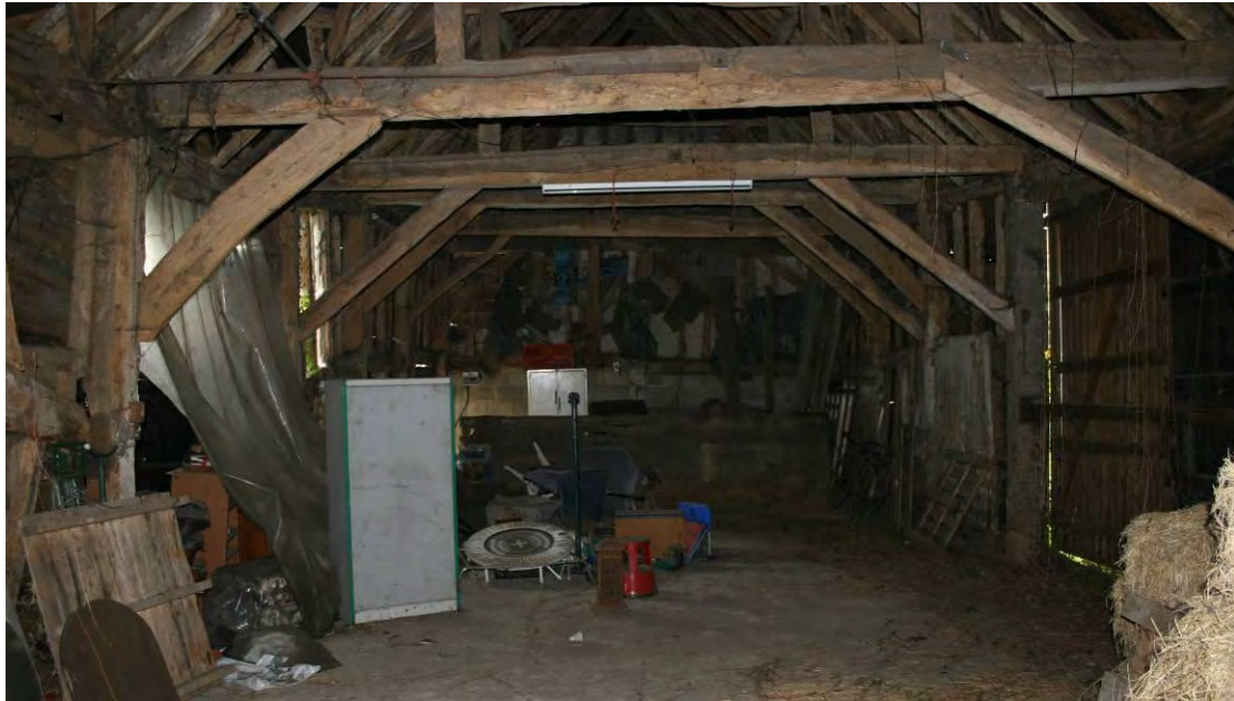
Looking E inside the Barn from the western end.
