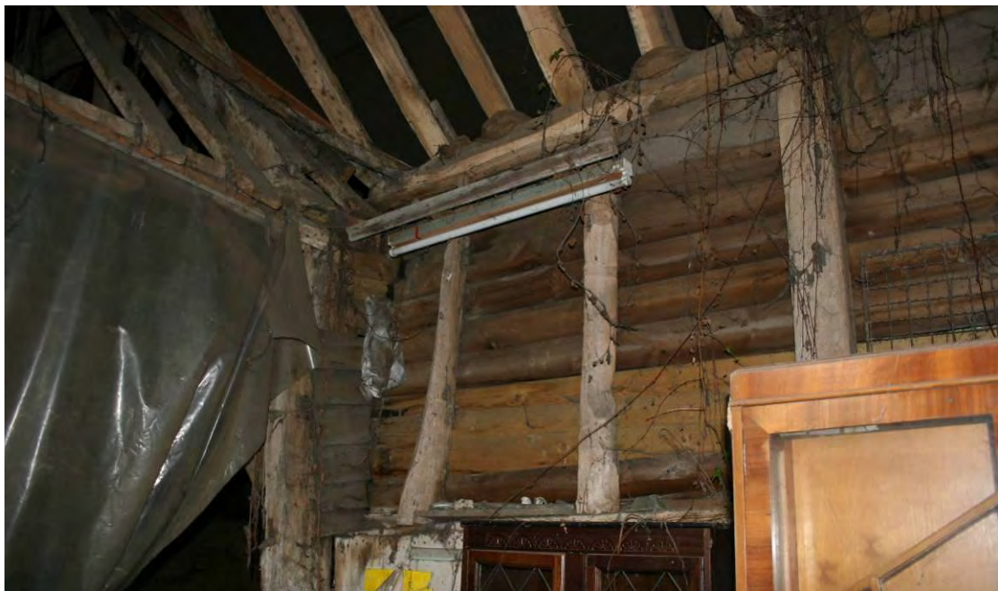
The frame visible on the western wall of the midstrey.
