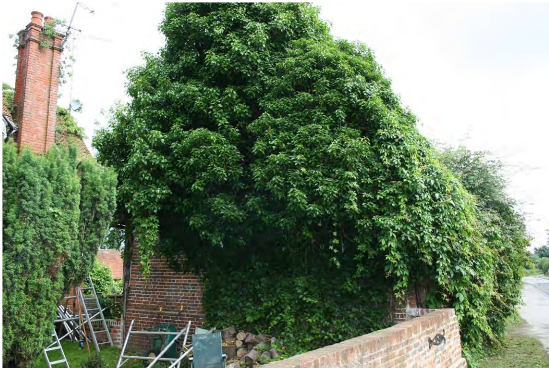
The western elevation of the Timber-framed Barn is made of brick.
