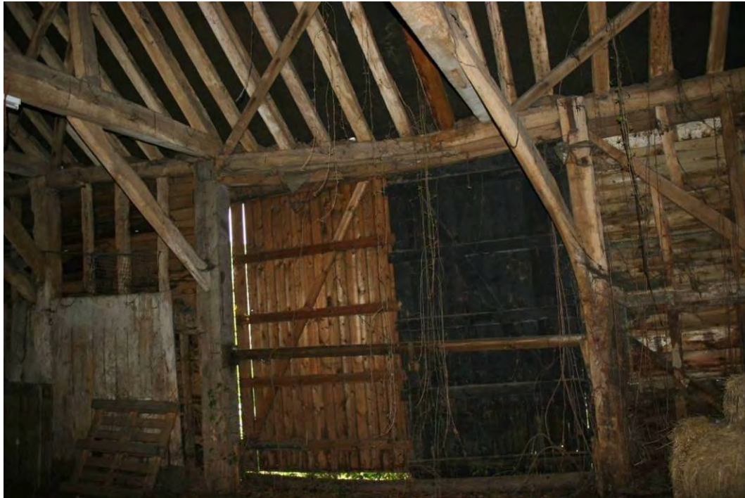
The trusses forming the midstorey. Note the displacement of the post. South doors.
