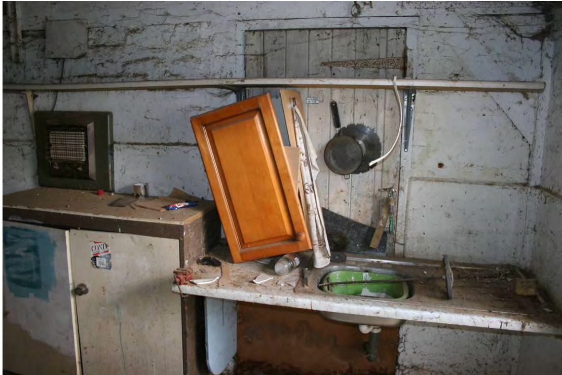
Processing and packing room. Sink and heater against the west wall.
