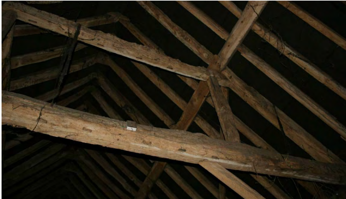
The frame of Truss 1 showing the mortices for an end wall. Looking SE.
