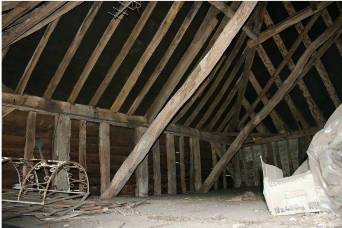
The grain loft in the top of the western extension. Looking SE.
