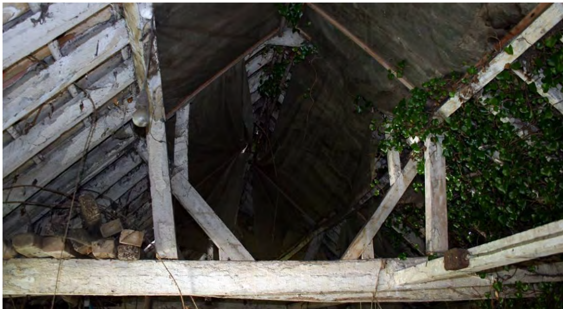
The roof structure in the southern half of the Workshop.
