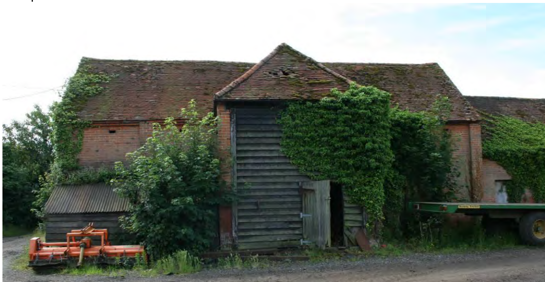
The northern elevation of the Brick Barn.
