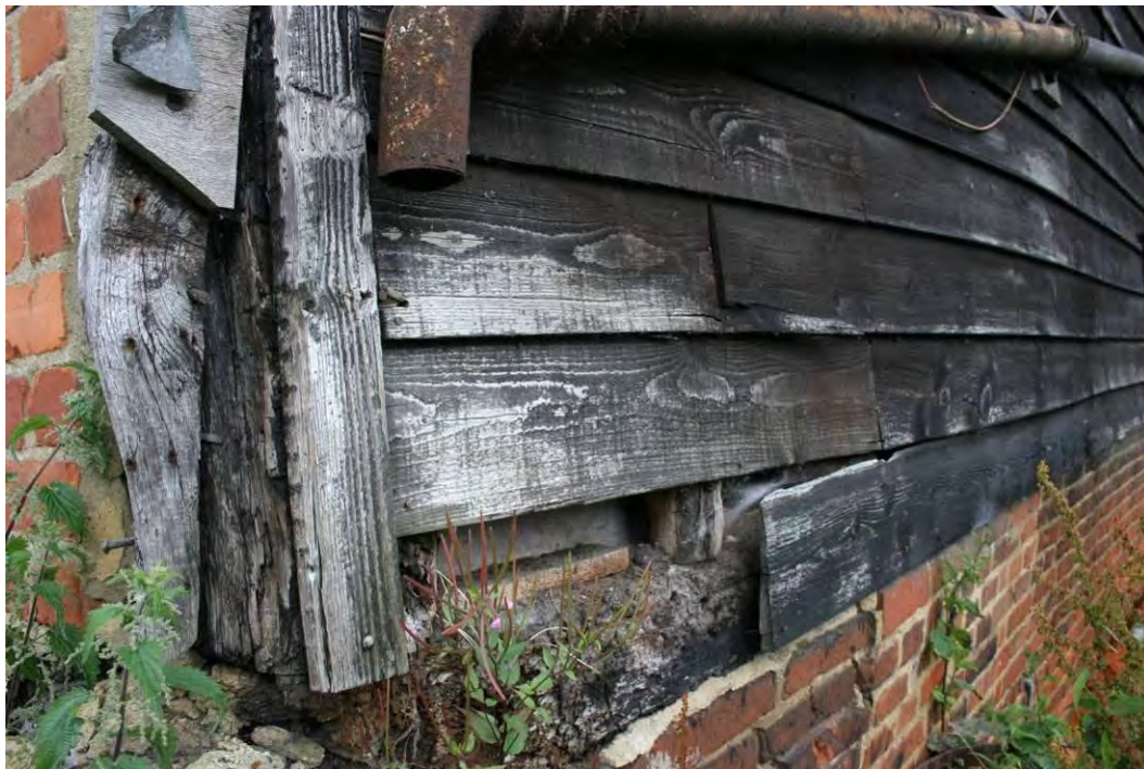
Detail of the C20th weather-boards and Tudor style bricks in the plinth.
