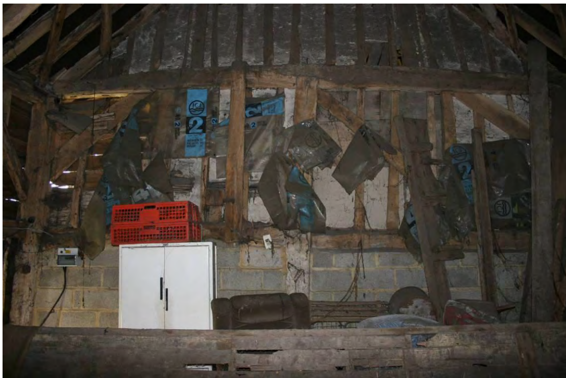
The upper section of the western wall frame.
