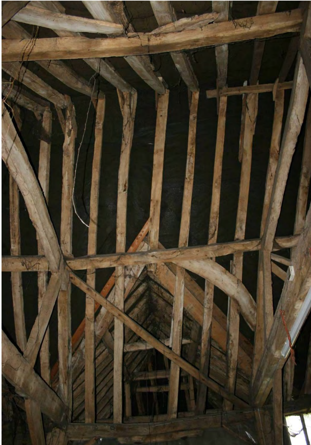
The northern side of the roof in Bay 3. Note the remnants of windbraces.
