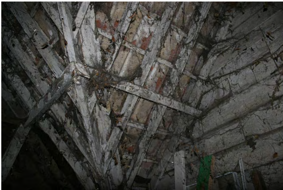
The roof structure in the corner room.
