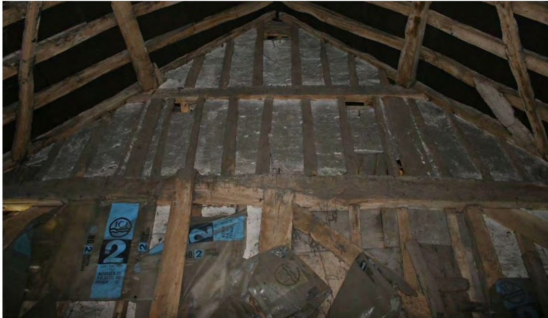
The upper section of the western wall frame.
