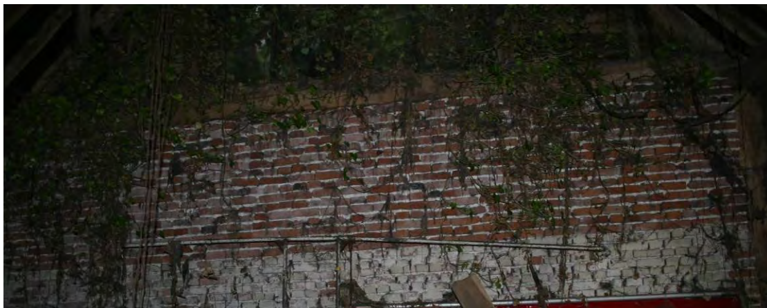
Detail of the brickwork from inside.
