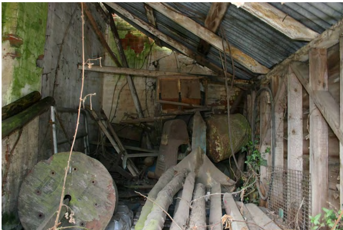
The interior of the timber shelter.
