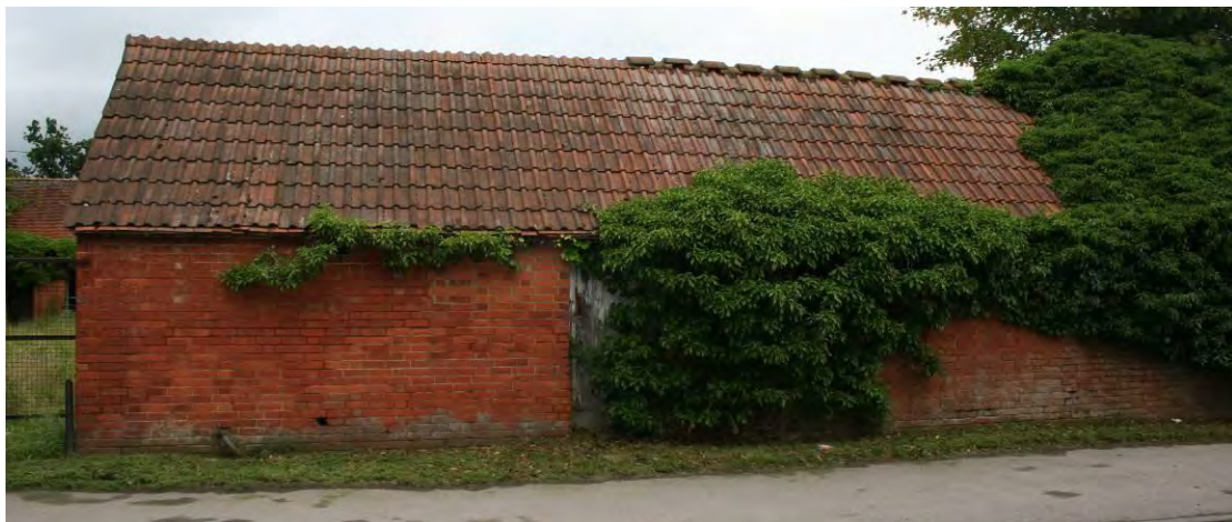
The southern elevation of the Processing Shed.
