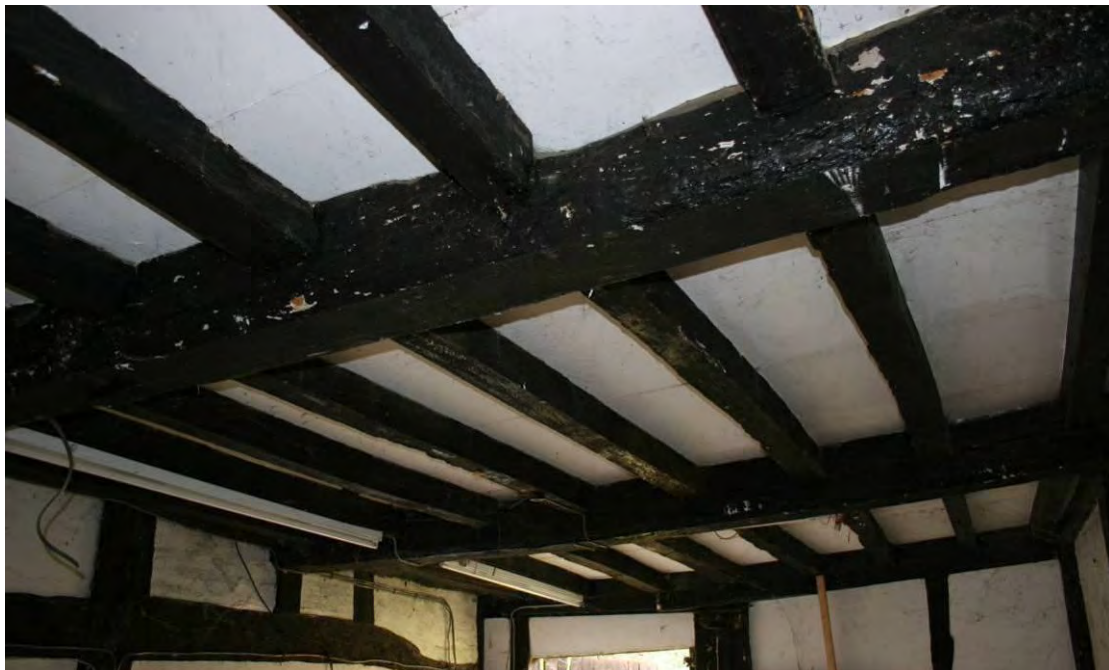
Framed granary floor in the western extension. Looking NW.
