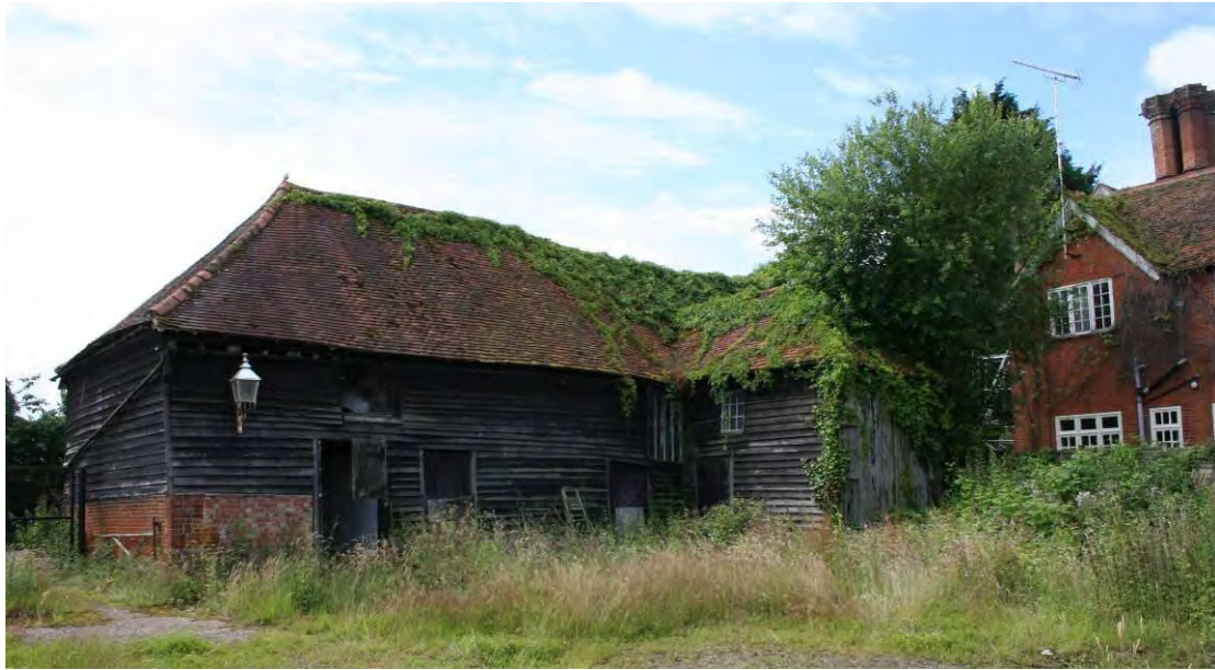
The Timber-framed Barn in context with the Farmhouse. Looking SW.
