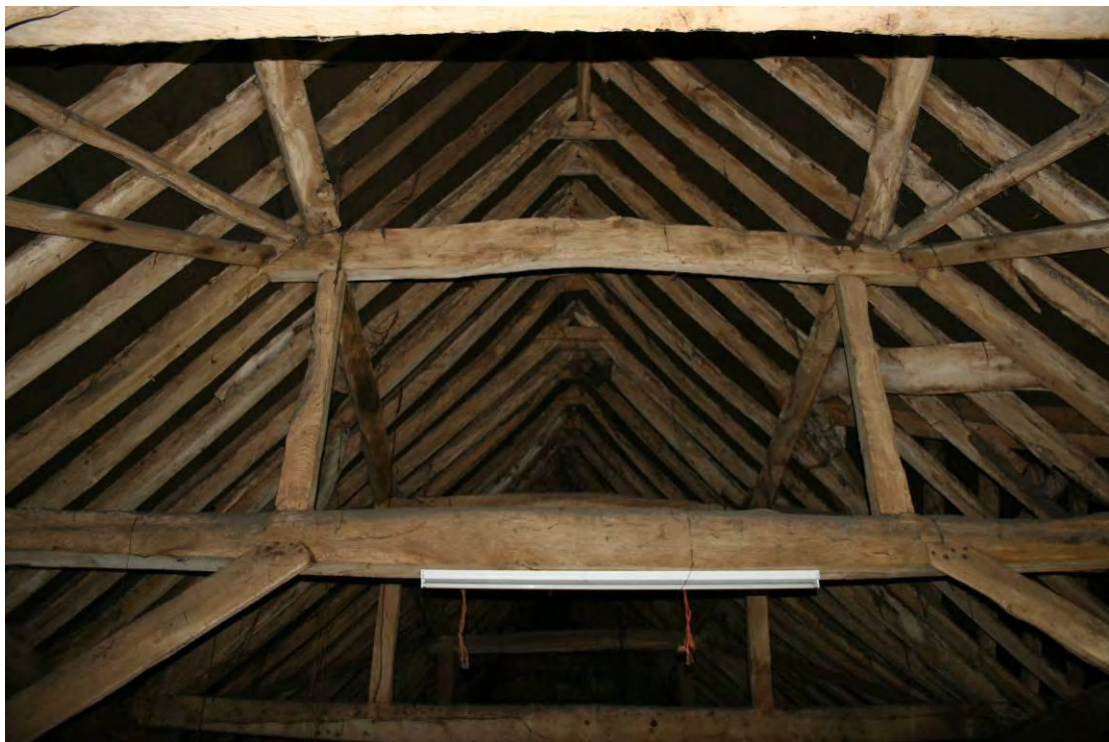
Truss 3 looking W.
