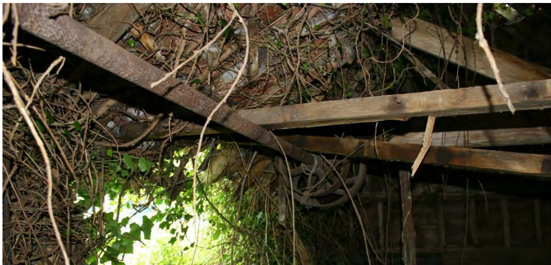
Machine drive shaft against the eastern wall.
