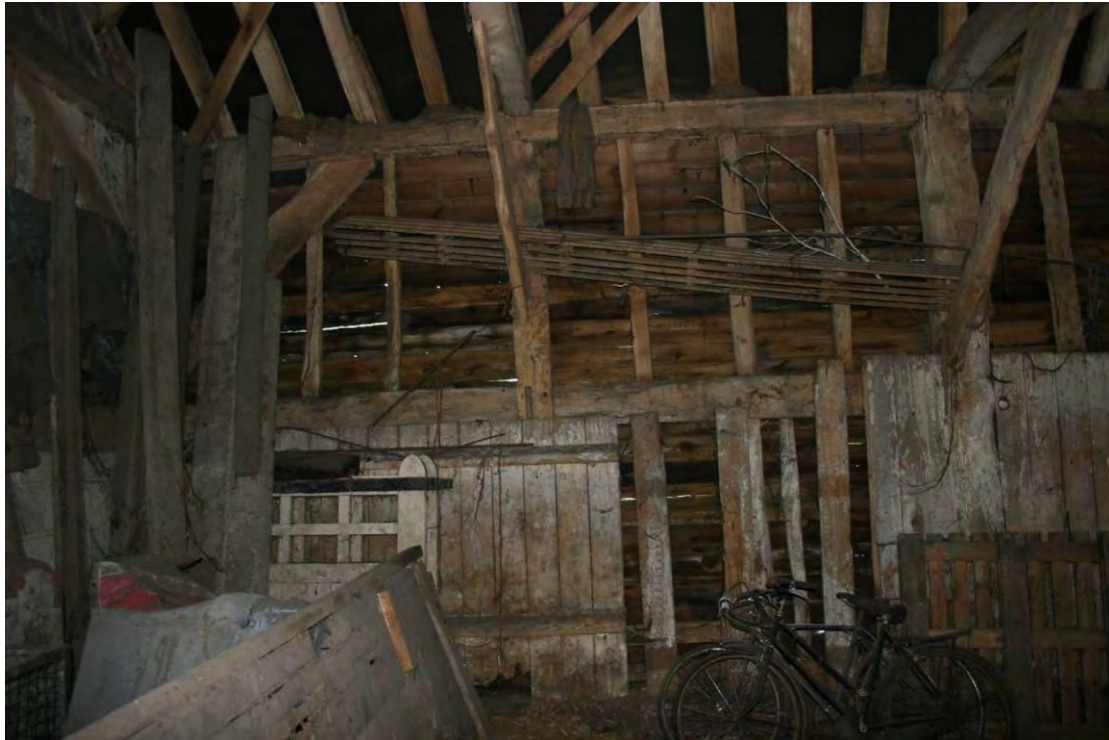
Wall frame in Bays 5 and 6, south side.
