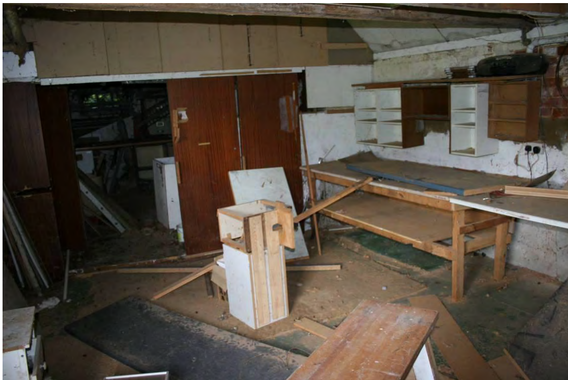
Processing and packing room. Looking SE.
