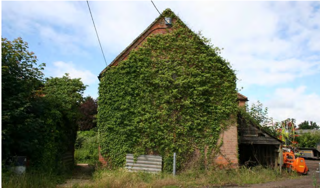
The eastern elevation of the Brick Barn.
