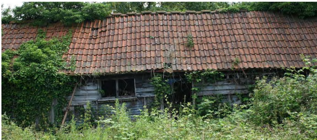
The southern half of the western elevation of the Workshop.
