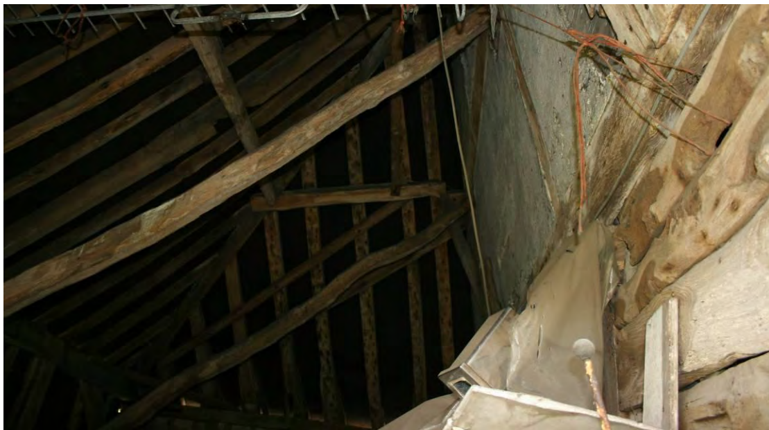
Looking up at the exterior wall of the Barn within the western extension.
