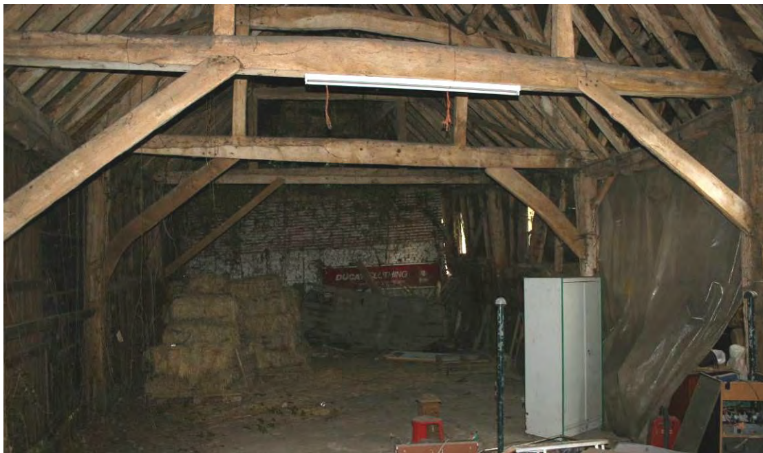
Looking W inside the Barn from the eastern end.
