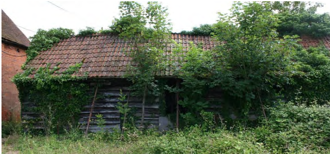
The northern half of the western elevation of the Workshop.
