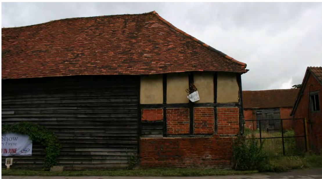
The southern elevation of the later extension to the Timber-framed barn.
