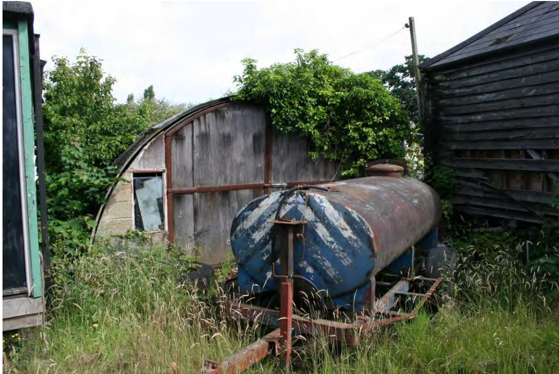
Storage Shed north of the farmyard.
