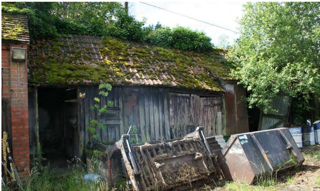
Detail of the exterior of the Tack Room and Garage Workshop.
