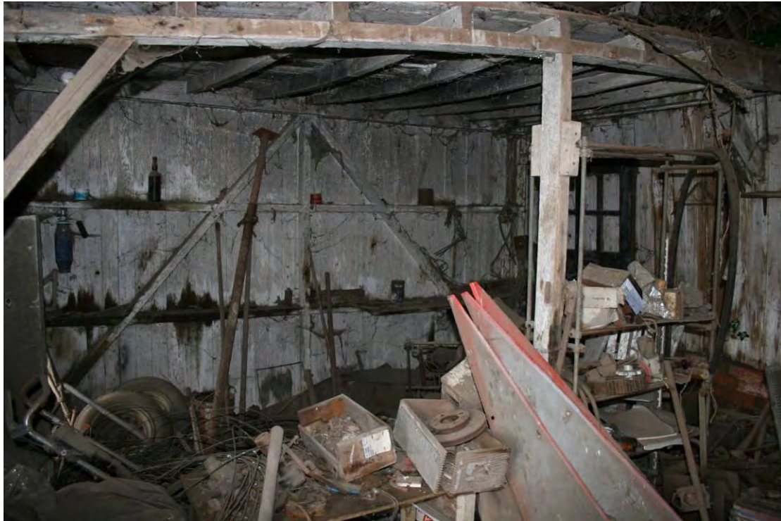
Looking W in the Garage Workshop. The partition is common with the Tack Room.
