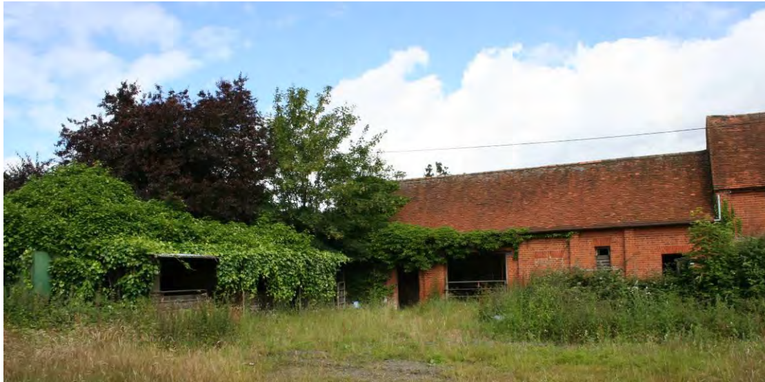
LC20th cow byre to the west of the farmyard. Looking NW.
