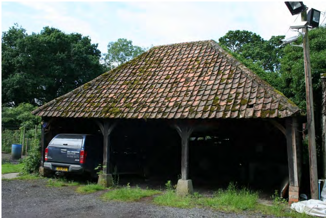
Shelter rebuilt in the 1960's. West of the farmyard. Looking W.
