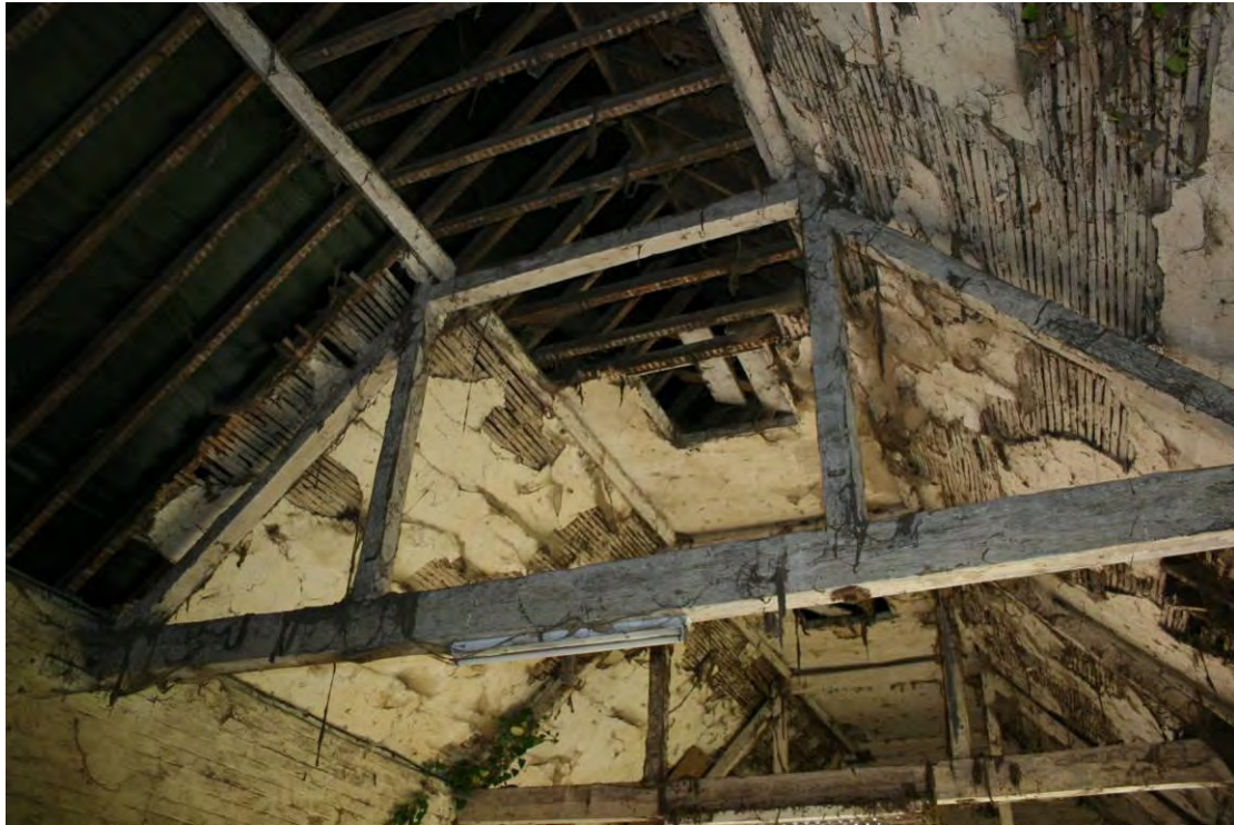
Detail of the roof structure. Looking NE.
