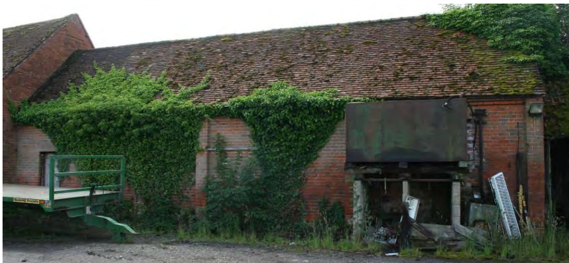
The Brick Stables northern elevation.
