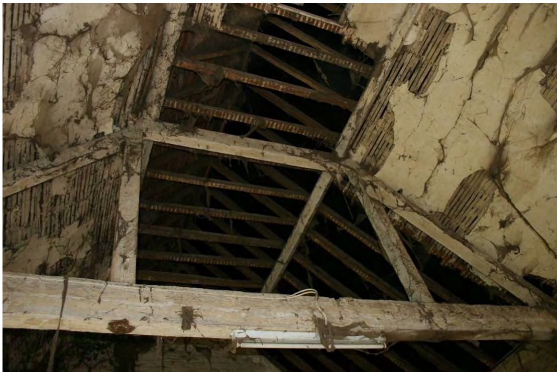
The roof is lath and plastered for insulation. Looking W.
