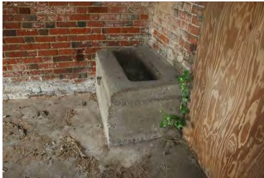
Concrete water trough.
