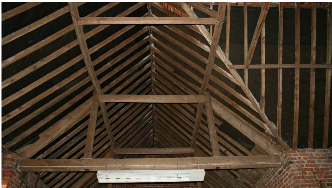
The roof mimics the style of the queen post roof in the Timber-barn.
