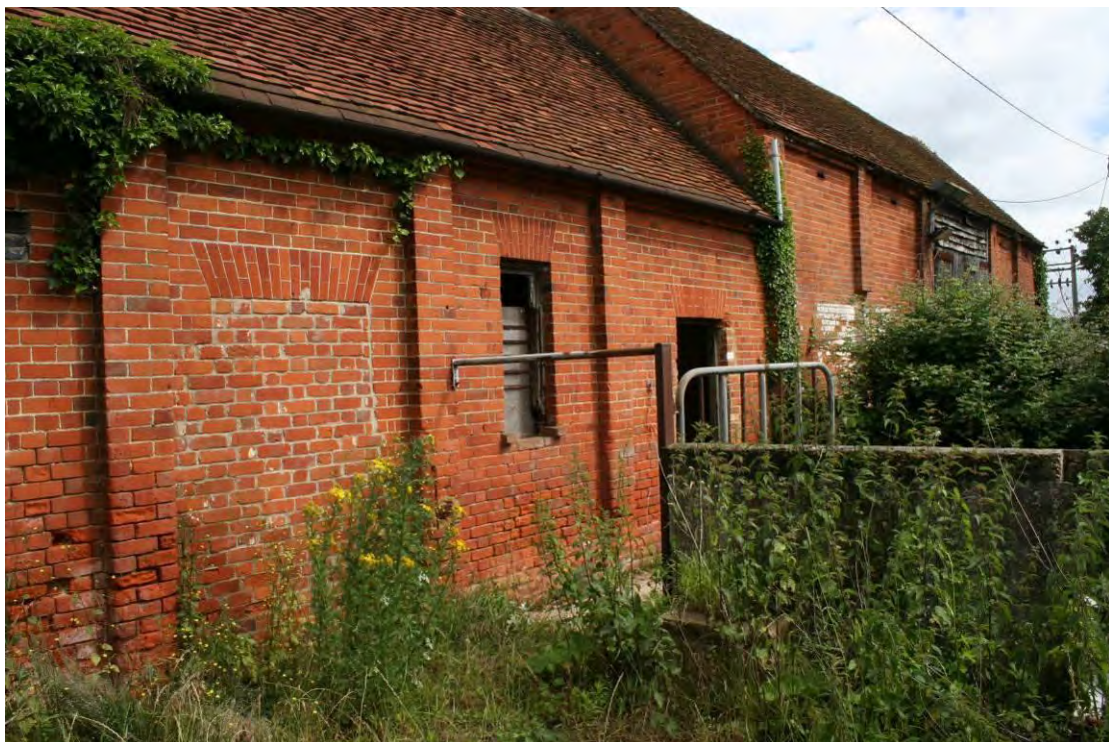
The southern elevation looking NE.
