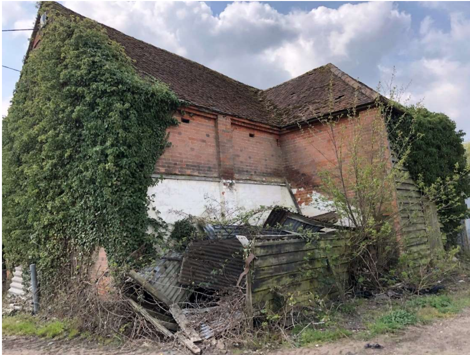
Figure 6: Exterior south elevation of unit 2
