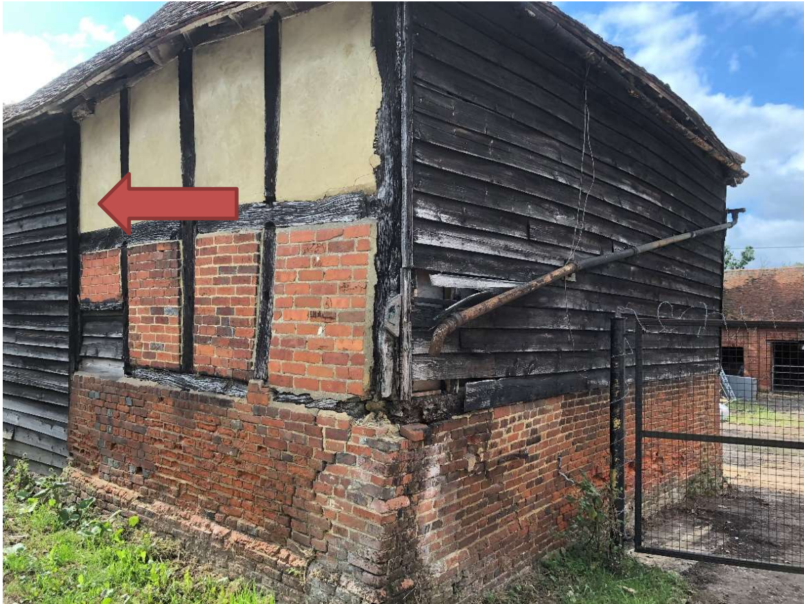
Figure 26: Unit 5 south east corner timber to brick junction detail
