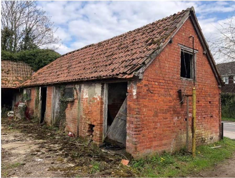
Figure 9: Courtyard view of unit 4
