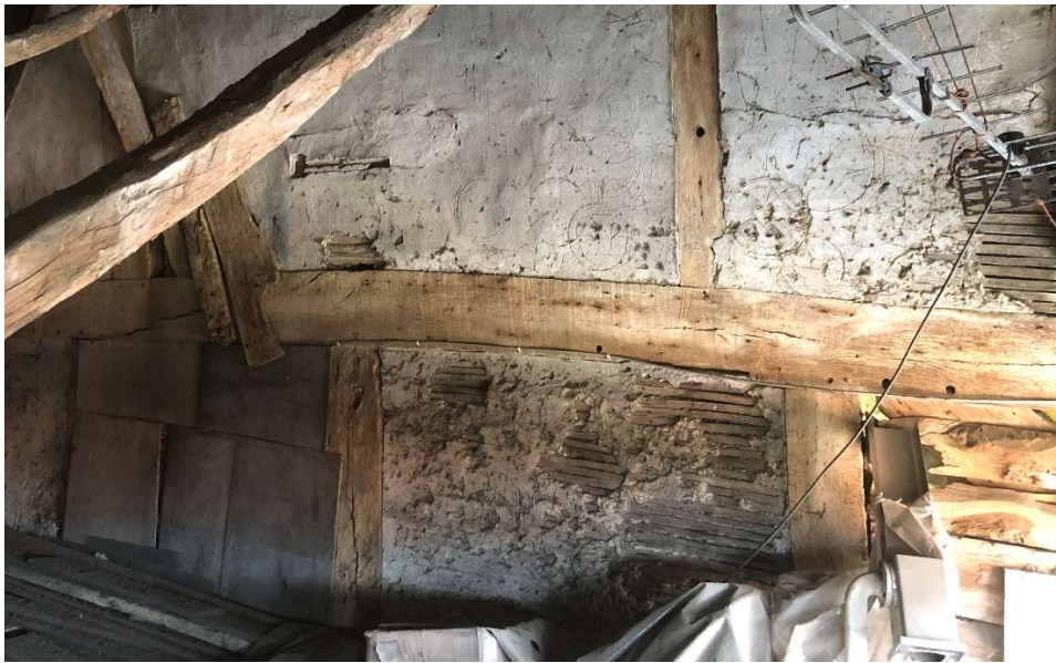
Figure 30: Photo of unit 5 bay 7 internal lime plaster
