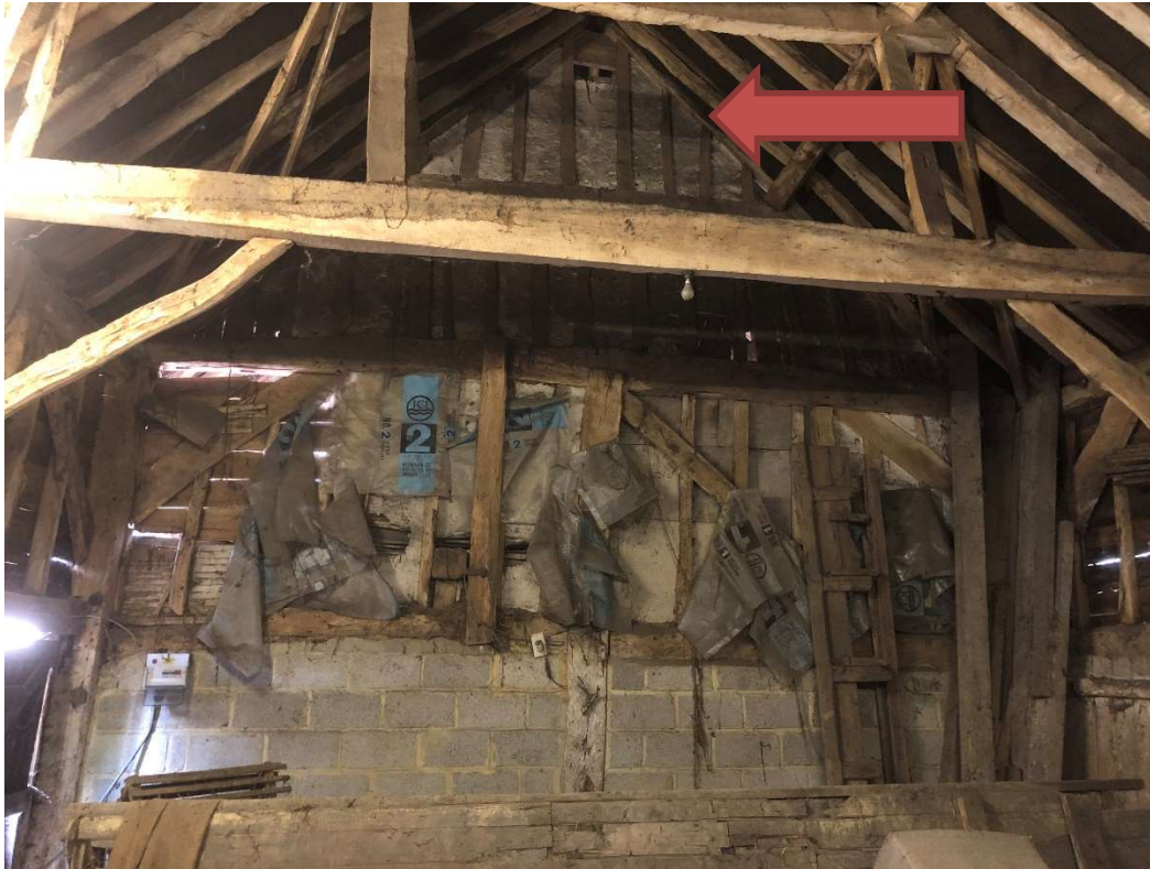
Figure 31: Photo of unit 5 Bay 7 internal wall to remain in situ
