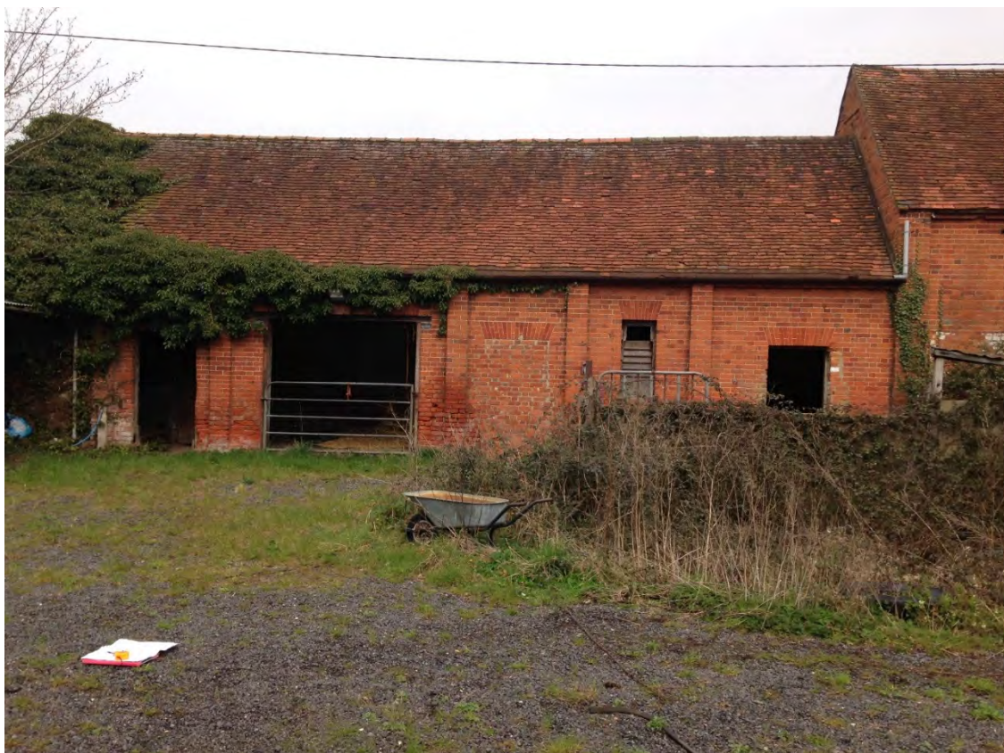
BUILDINGS 'D' & 'E'
