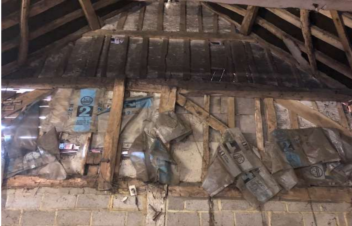
Photo 23 – Bay 6 eastern hay loft elevation
