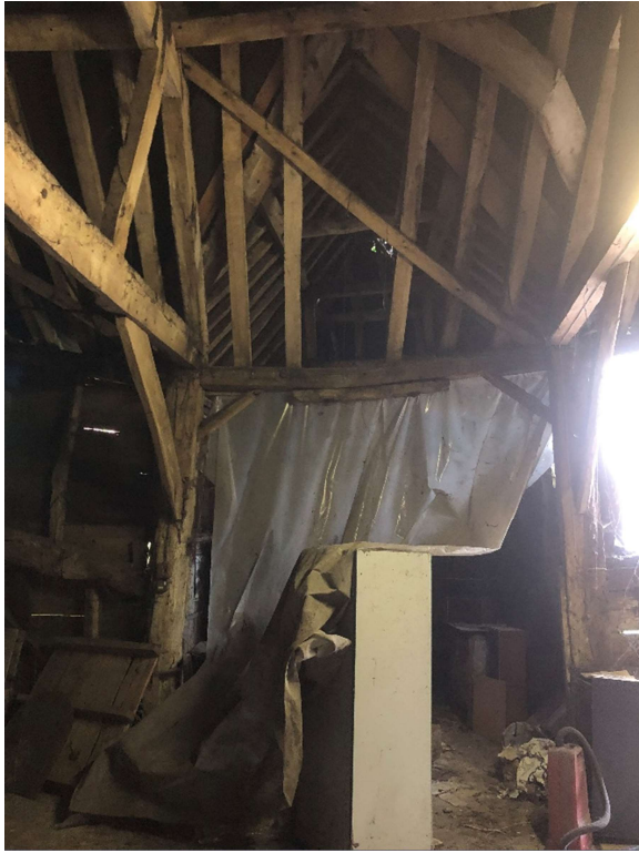
Photo 15 – Porch facing North from main barn
