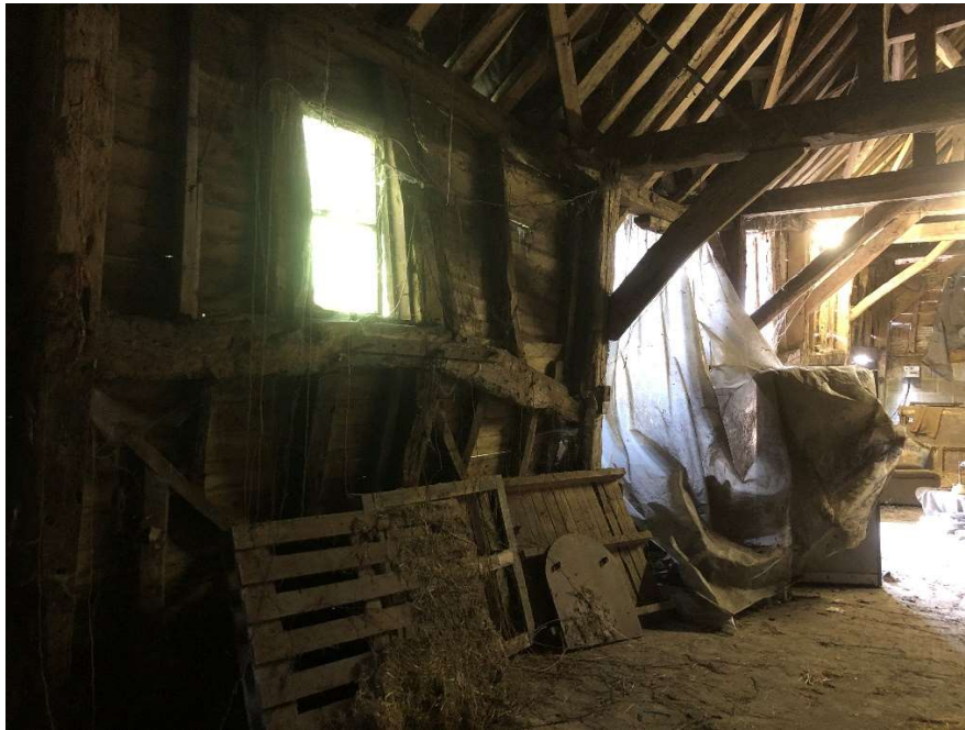
Photo 21 – Bay 2 wall section facing northeast
