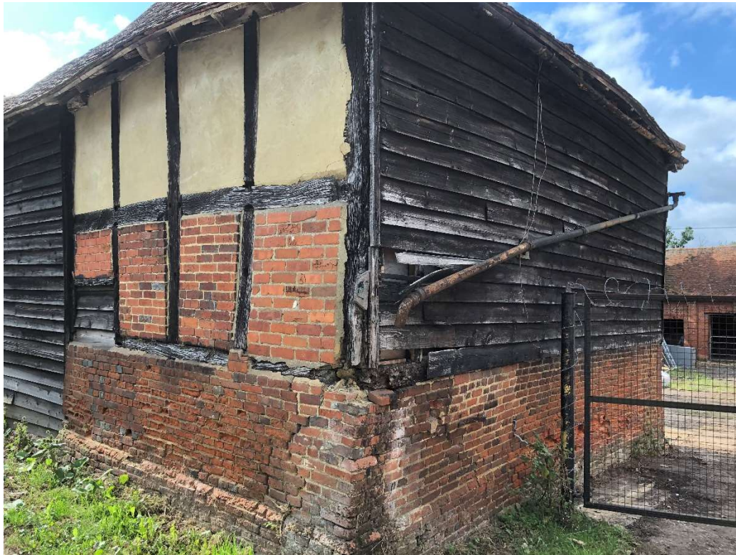
Photo 3 – South-east corner elevation
