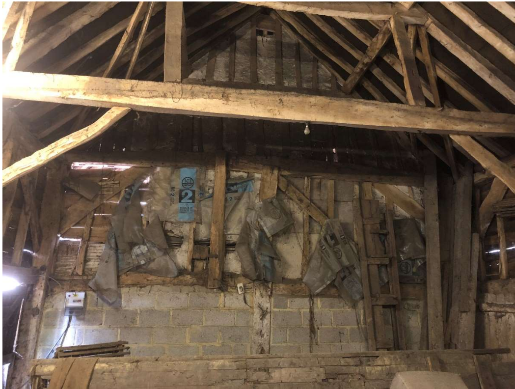
Photo 11 – Bay 6 facing East
