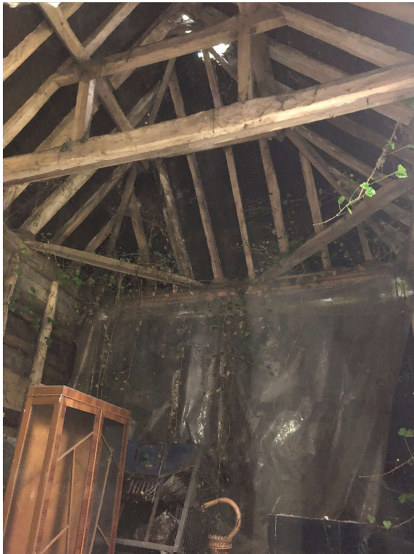
Photo 16 – Porch roof bay facing North
