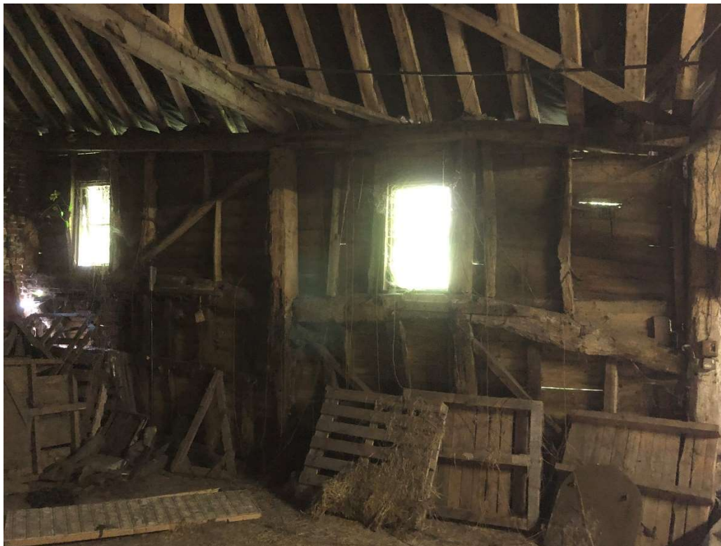
Photo 14 – Bay 2 North wall panel
