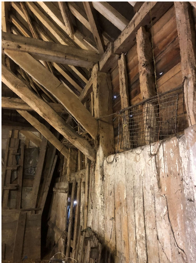
Photo 22 – Bay 4 facing southeast detail of wall section showing additional wall cladding
