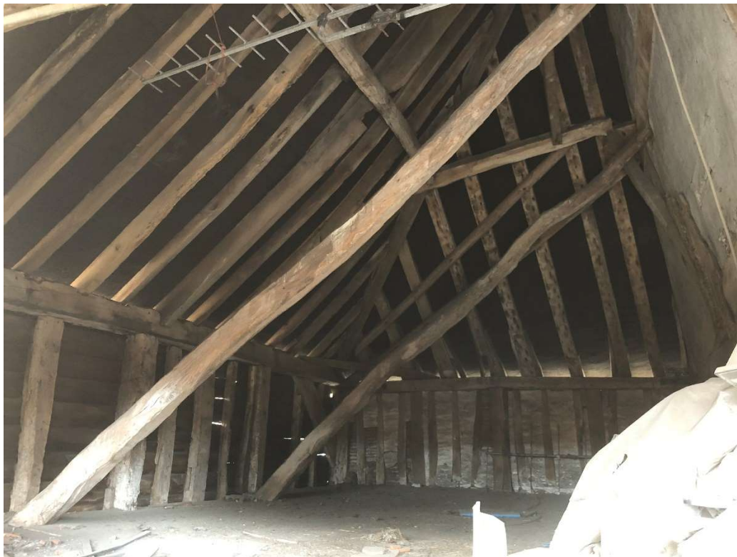
Photo 8 – Roof Bay 7, hayloft first floor
