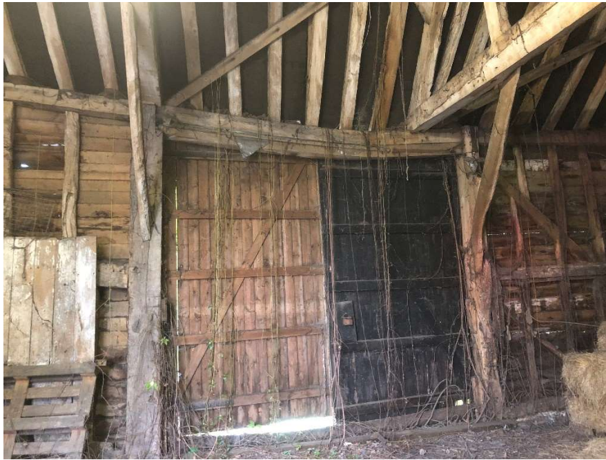
Photo 17 – Bay 3 - Main southern barn doors
