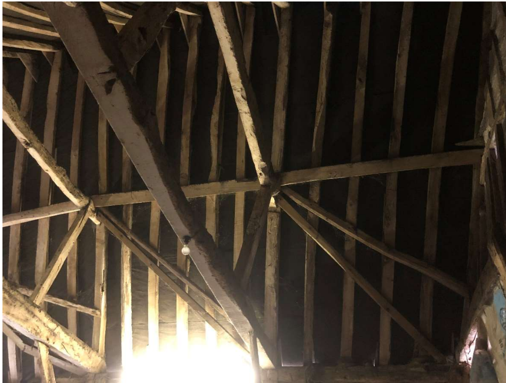
Photo 13 – Roof Bays 4 and 5 facing North
