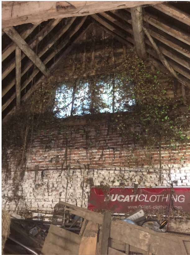
Photo 19 – Bay 1 – Window in brickwork to west elevation
