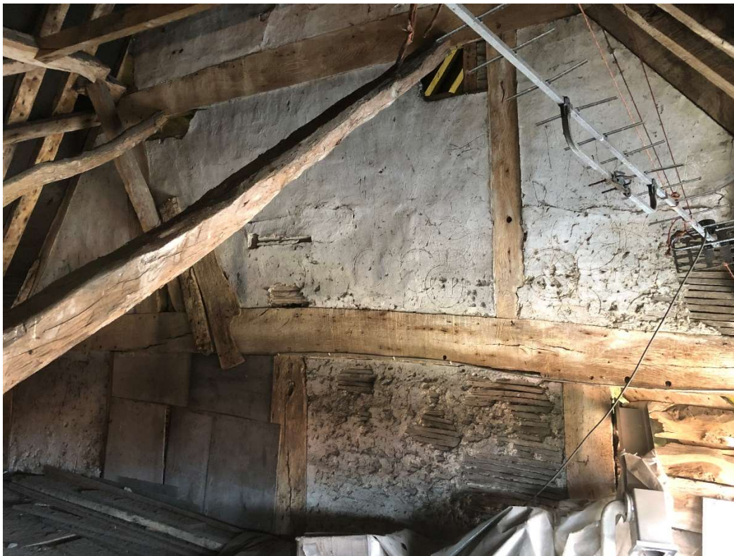
Photo 10 – Roof Bay 7 wattle and daub panels
