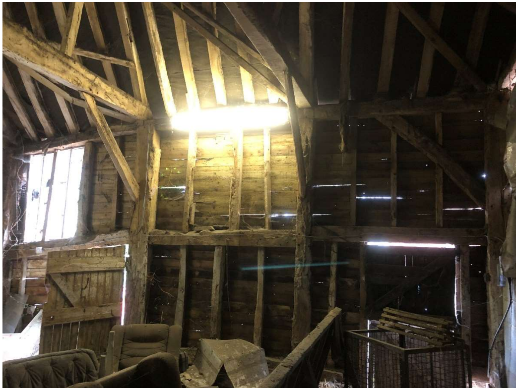
Photo 12 – Bay 5 Northern wall panel
