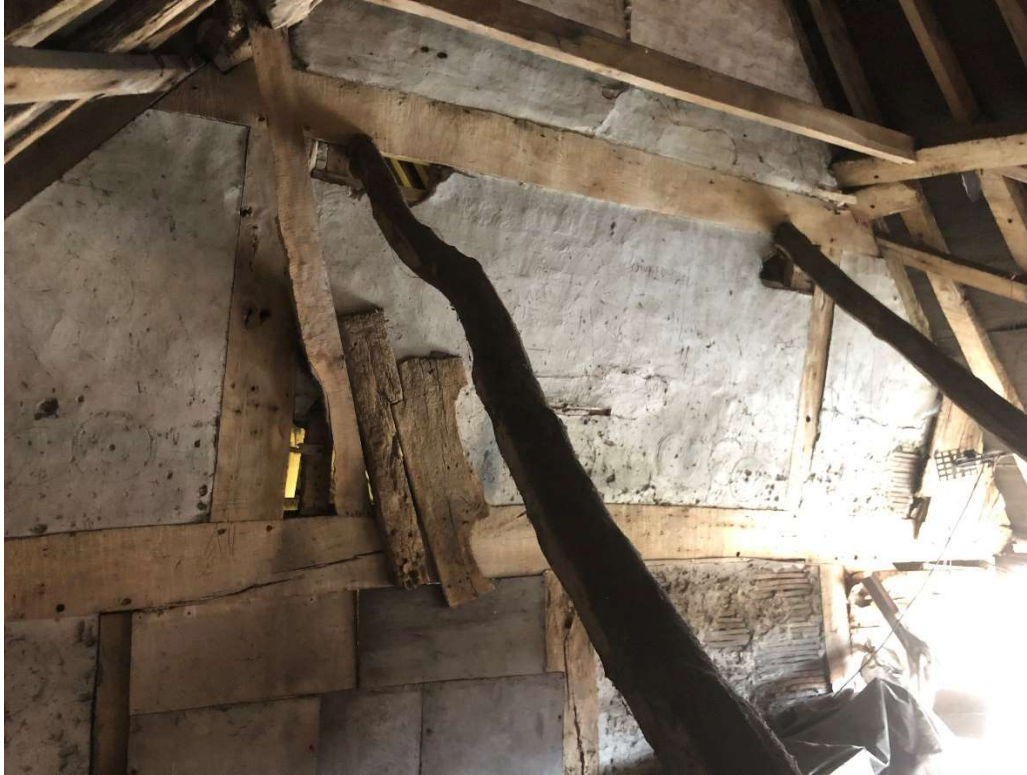
Photo 9 – Roof Bay 7 wattle and daub panels
