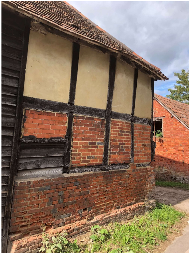
Photo 2 – South-eastern corner panels in timber frame
