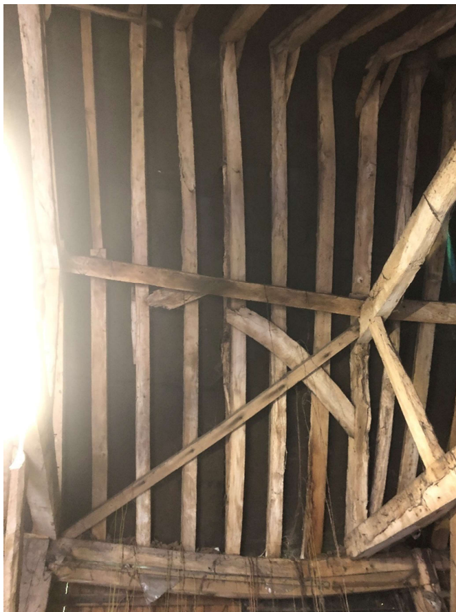
Photo 18 – Bay 3 Roof section facing south
