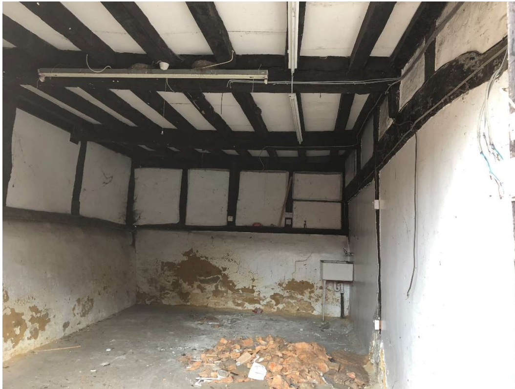
Photo 7 – Bay 7, hayloft ground floor
