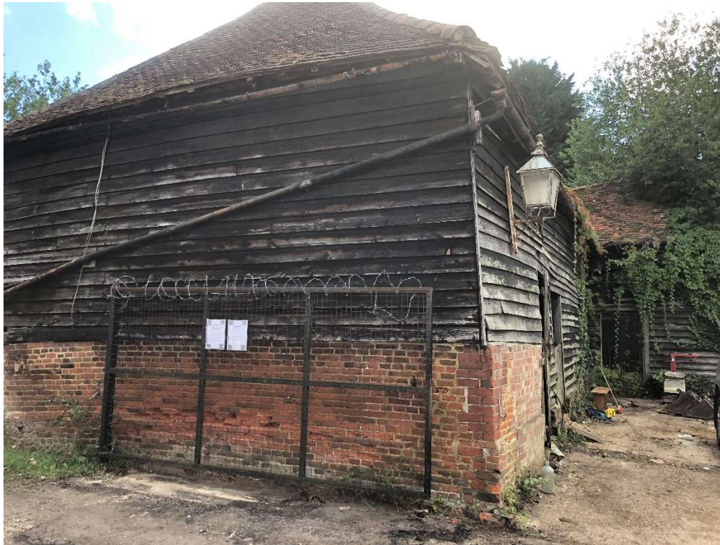
Photo 5 – East and Northern elevations
