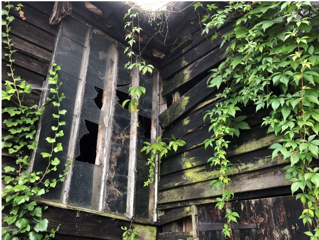
Photo 6 – Window to North elevation Bay 4
