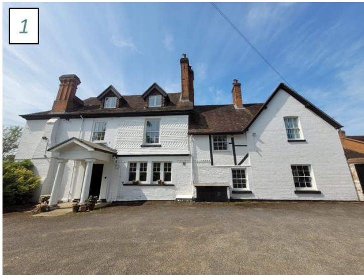
Figure 6: Photos of the site
