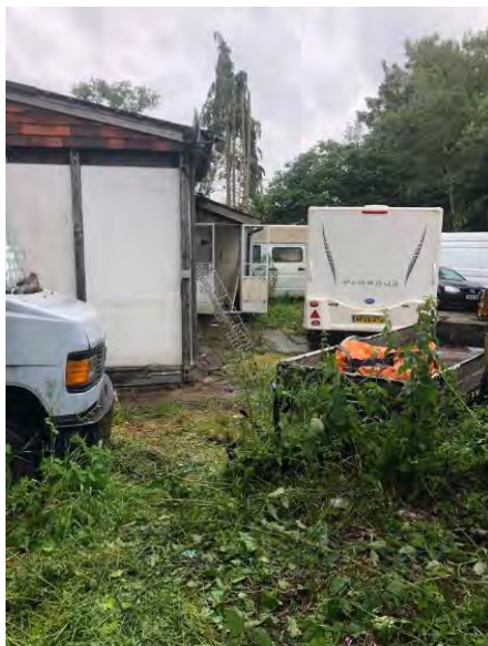
Photograph 6: south-western corner of the building (facing north-east)
