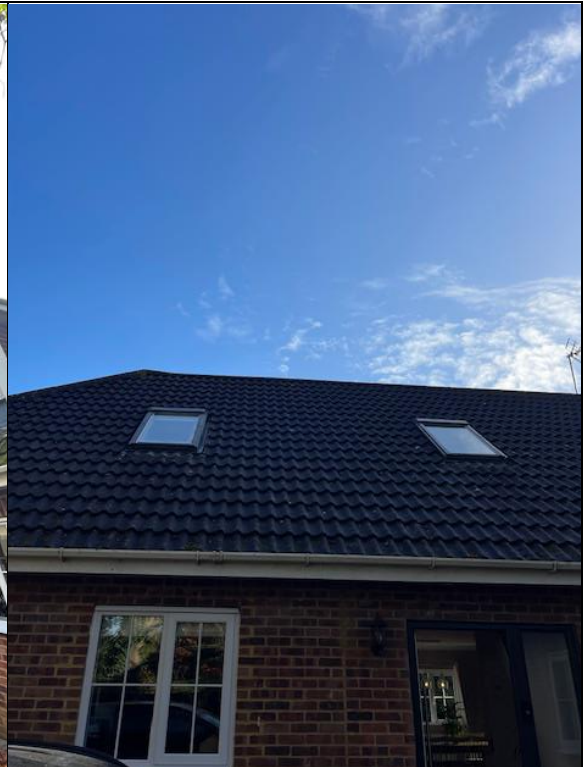
Photograph 10: Interlocking roof tiles.
