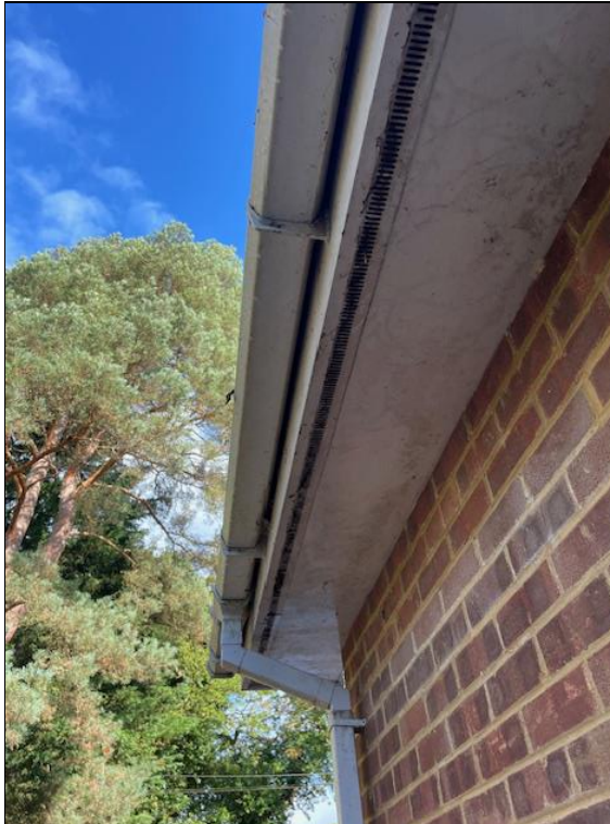
Photograph 13: No visible gaps around the soffits.
