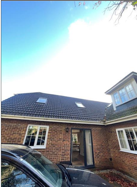
Photograph 9: Interlocking roof tiles.
