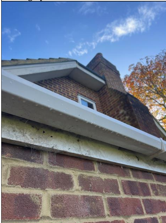
Photograph 7: uPVC guttering.
