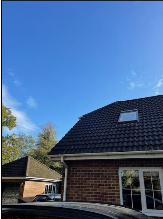
Photograph 11: Interlocking roof tiles.
