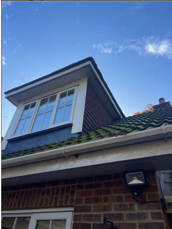
Photograph 3: Dormer window with hanging tiles.
