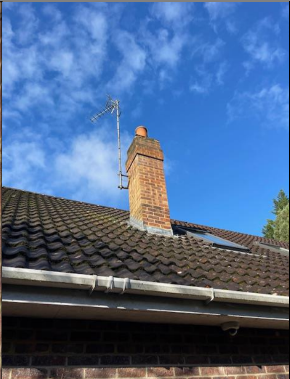
Photograph 18: Side elevation-interlocking roof tiles.
