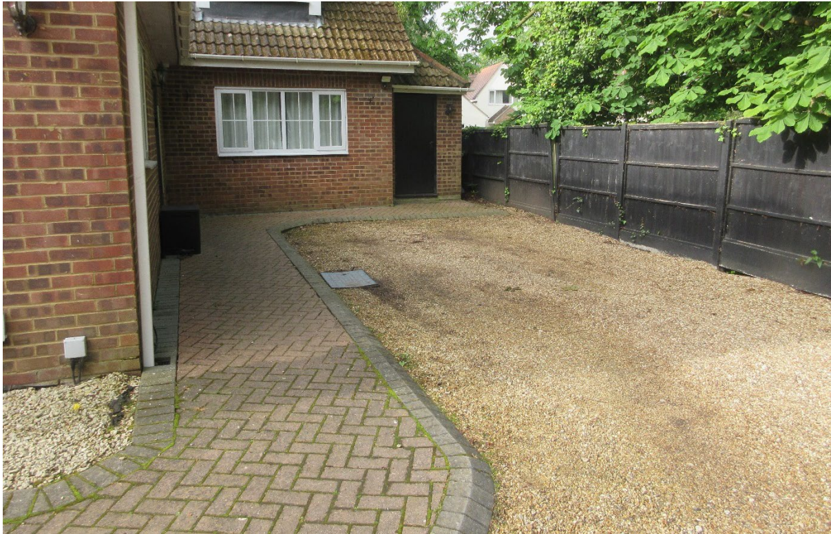
Photograph 2: Showing the existing ground conditions in the location of the proposed extension, note the compacted gravel surface, 1.25m wide brick paved path and the manhole.
