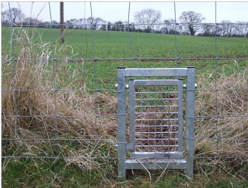
Plate 1: Example of a galvanized steel mammal gate within a deer fence that will be installed within the fence line.
