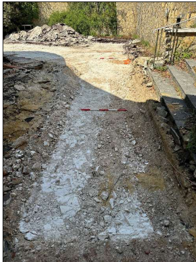
Plate 2: Trench 1. View to the northwest with foundation cut for staircase [1005] to the right of the image. 1m scale.
