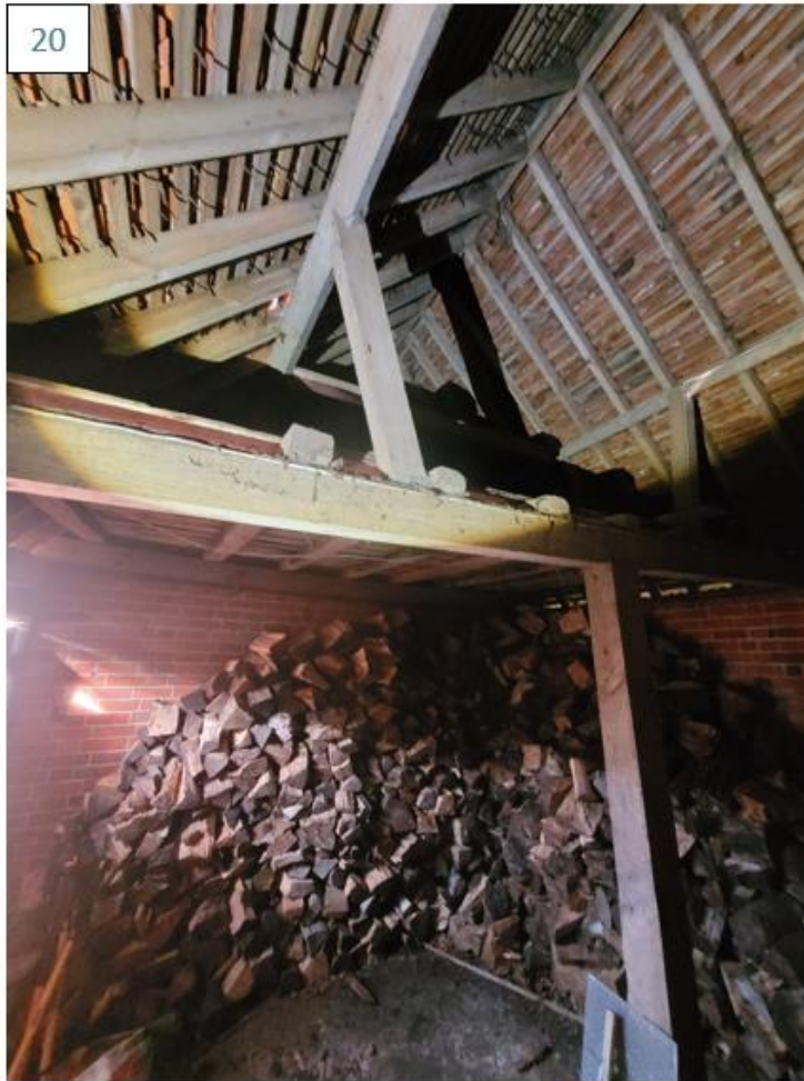
20: Wood store with unlined roof above. 21: Potting shed with chicken wire above.
