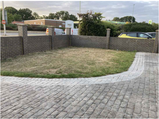
Existing Wall and Parking Area
