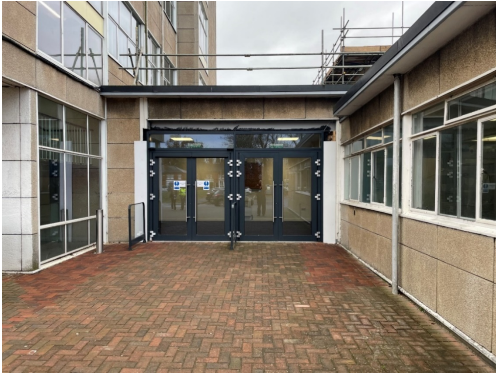
New Glazed Doors at St Crispin's School, Wokingham
