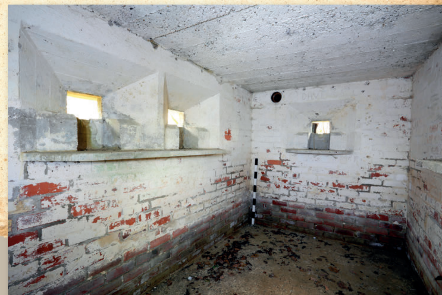
Pillbox interior with eastern double loophole, vent and southern wall
