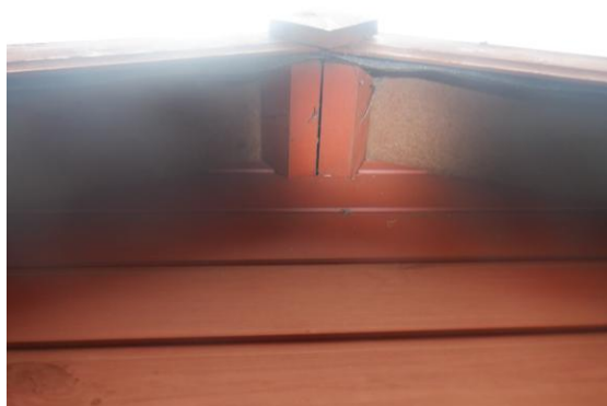
Photograph 5. Gable sealed to internal roof lining (Outbuilding 2).
