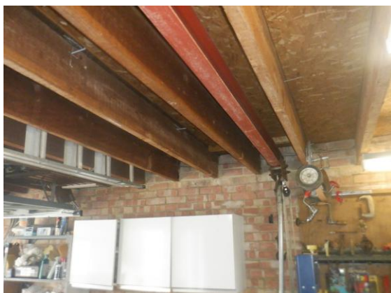
Photograph 15. Chipboard roof sealed to the internal brickwork walls (Garage).
