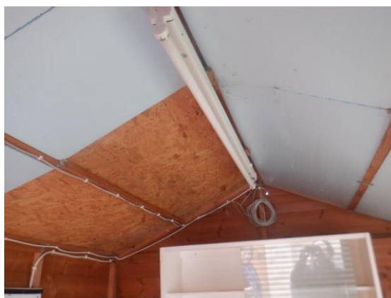
Photograph 11. Timber panel walls and chipboard roof fully sealed (Outbuilding 4).
