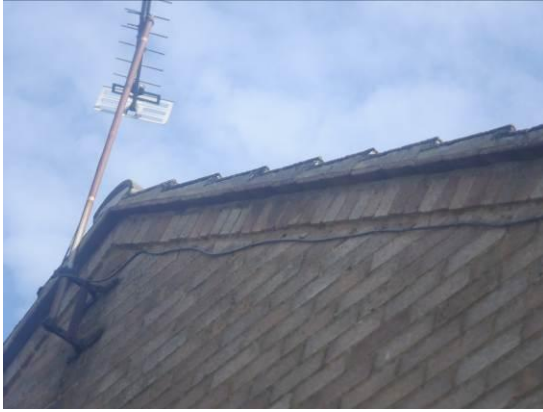
Photograph 5. Complete tile end mortar at north western side gable
