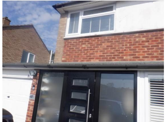
Photograph 8. Tightly fitted bitumen felt above the front porch and garage.
