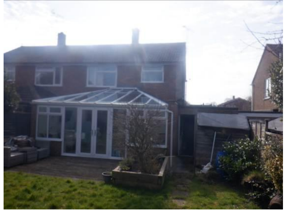
Photograph 2. Rear of property viewed from south.
