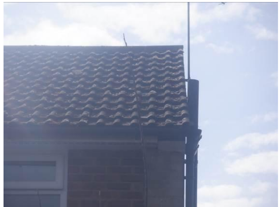
Photograph 4. Rear extension roof (rear elevation).
