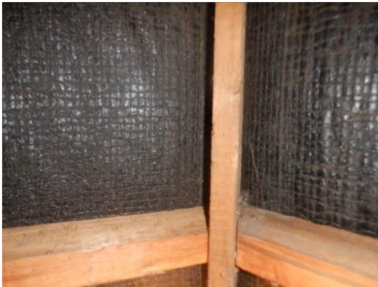
Photograph 11. Lightly cobwebbed ridge and intact bitumen felt.
