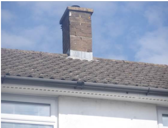
Photograph 3. Main roof (front elevation).
