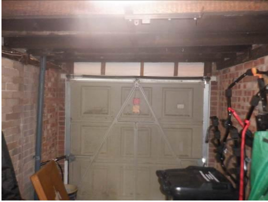
Photograph 17. The interior of the garage.
