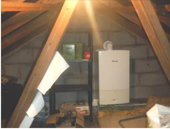
Photograph 9. Main roof void.
