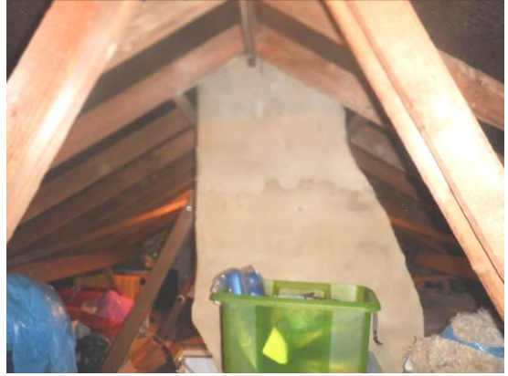
Photograph 10. Cement covered chimney
