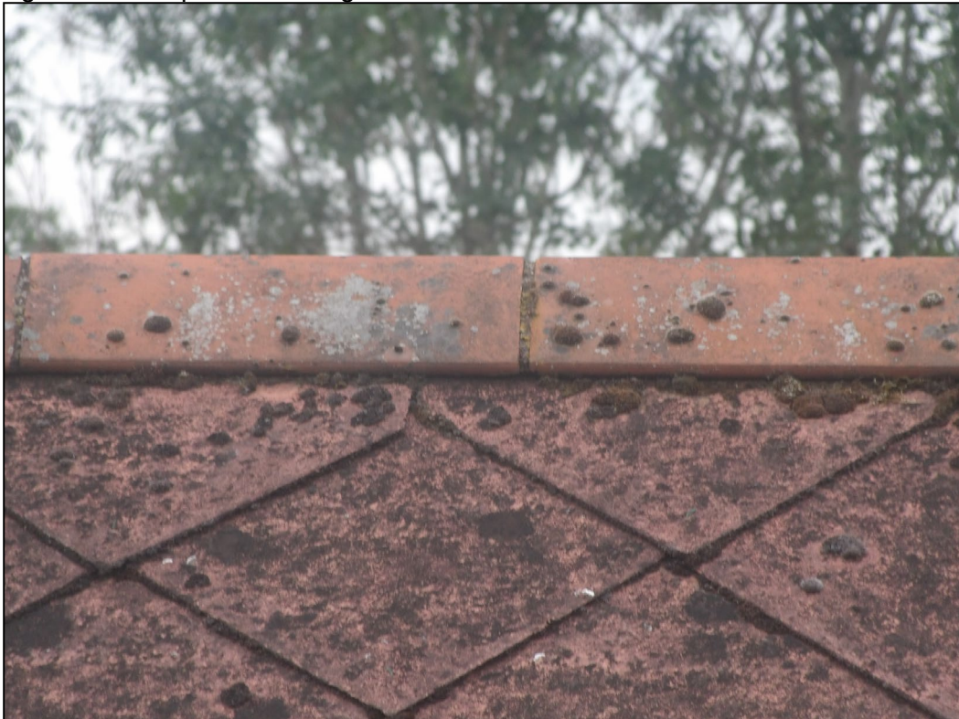
Figure 6. Example sealed ridge tiles. 37 Hatch Ride, Crowthorne. 27.08.24
