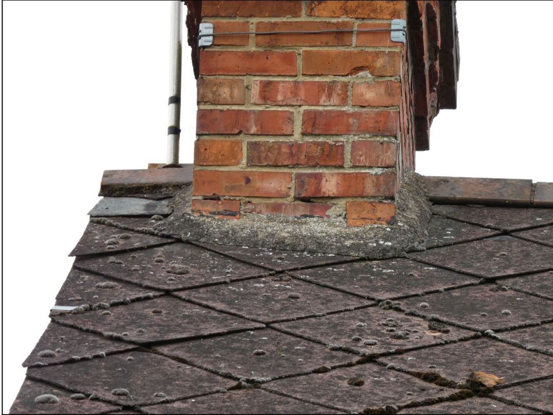
Figure 7. Example of cement around the chimney stacks. 37 Hatch Ride, Crowthorne. 27.08.24
