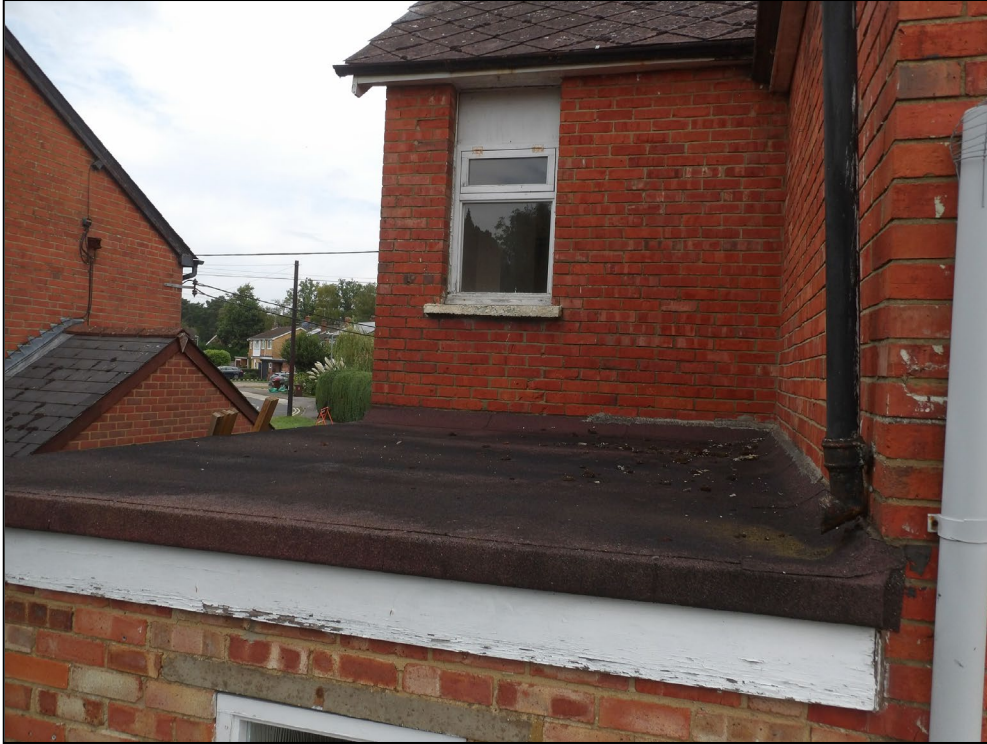
Figure 9. Bitumen covering on rear single storey extension. 37 Hatch Ride, Crowthorne. 27.08.24
