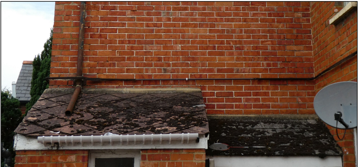
Figure 10. Roof tiles of 'lean-to' style extensions. 37 Hatch Ride, Crowthorne. 27.08.24
