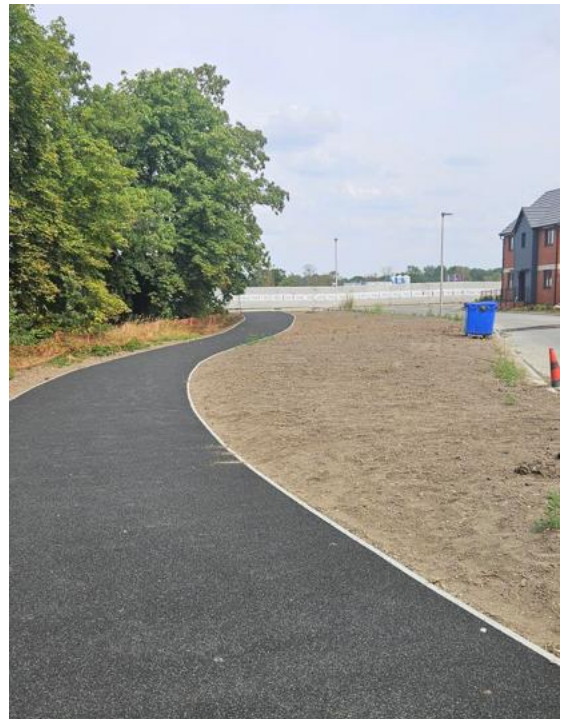
North of District Centre 3.5m Shared Path
