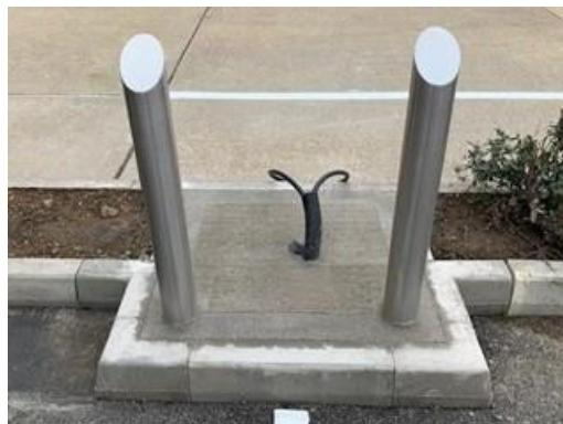
**FIGURE 5: STAINLESS STEEL PROTECTION POSTS**
