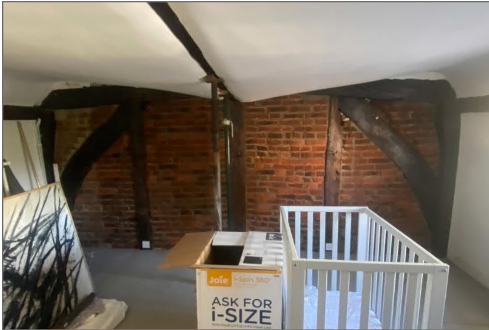
Image 09: View of brickwork to First Floor West gable
