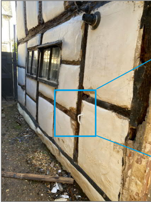
Image 05a: View of West gable
