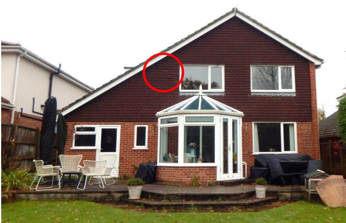
Image 3 – South facing elevation of the property where gaps of accessible proportions to offer likely shelter/access opportunities for bats were observed
