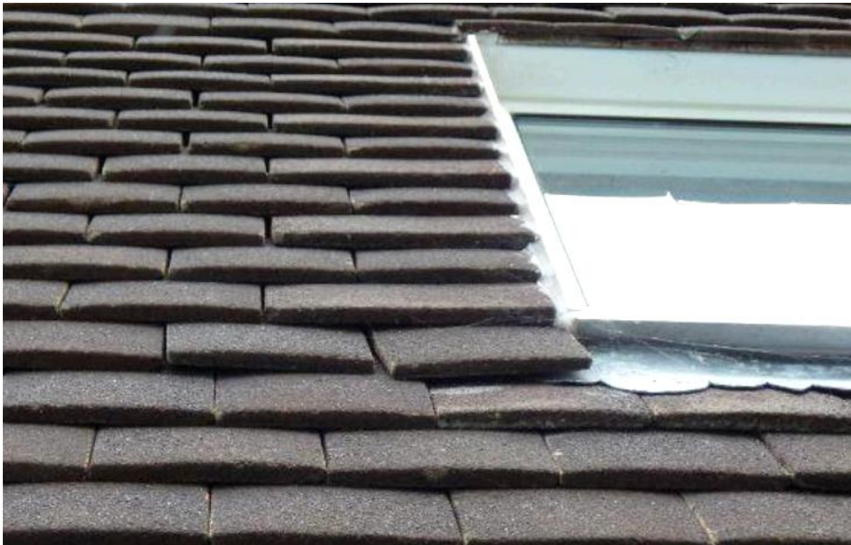
Image 2 – Close view of the North facing vertical hanging tiles which has demonstrated minor gaps of potential value to bats within
