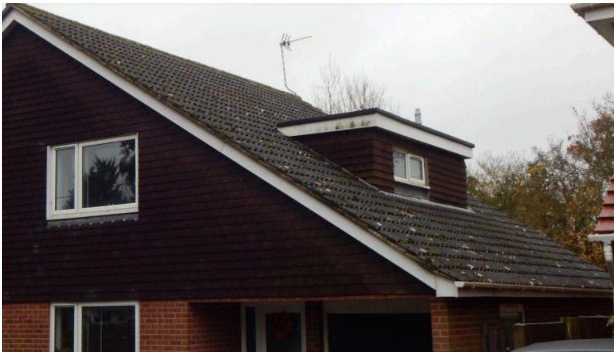
Image 6 – West facing elevation of the property
