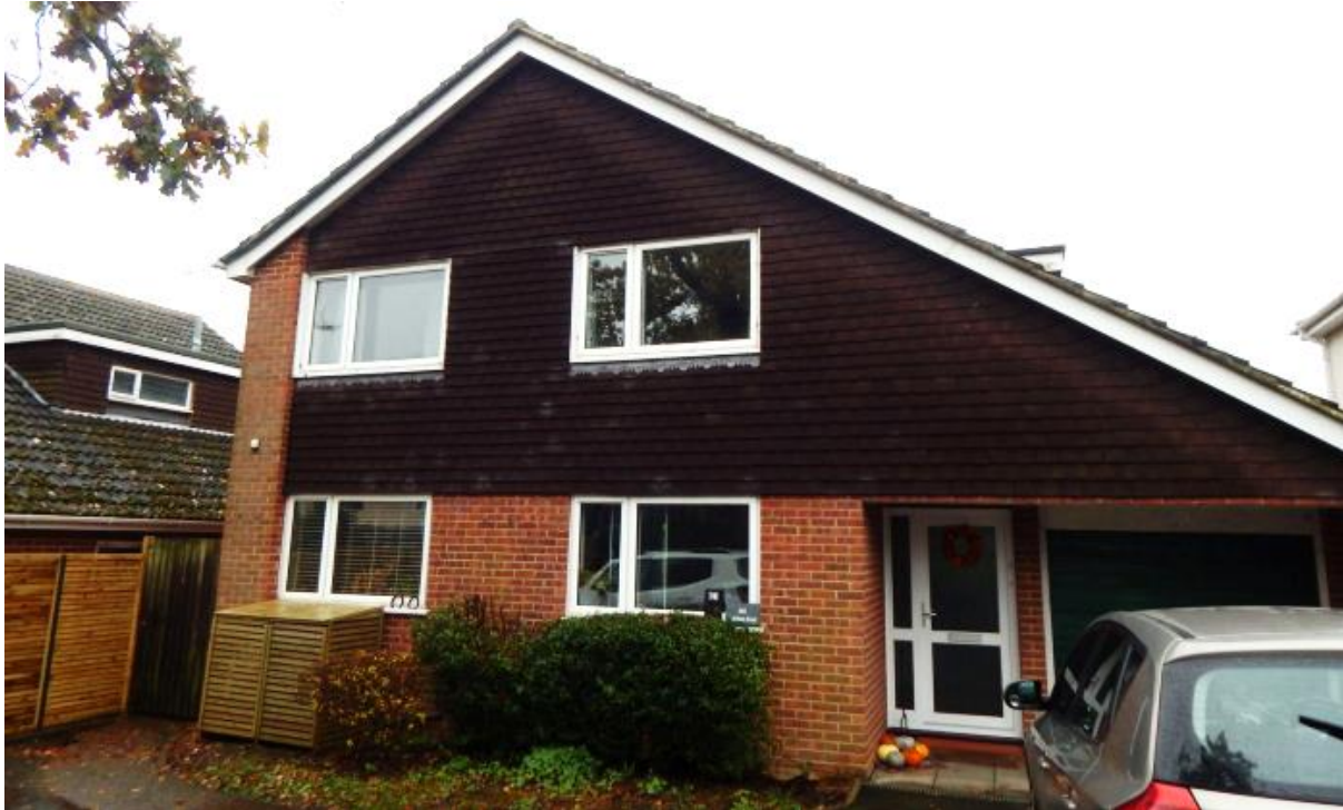
Image 1 – North facing elevation of the property
