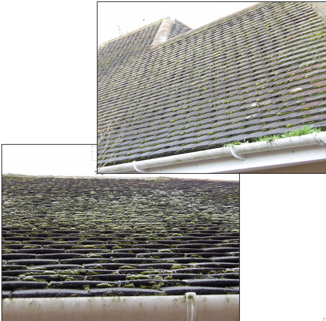
Figure 4. Example of roof tiles. 108 Reading Road, Woodley. 10.01.25
