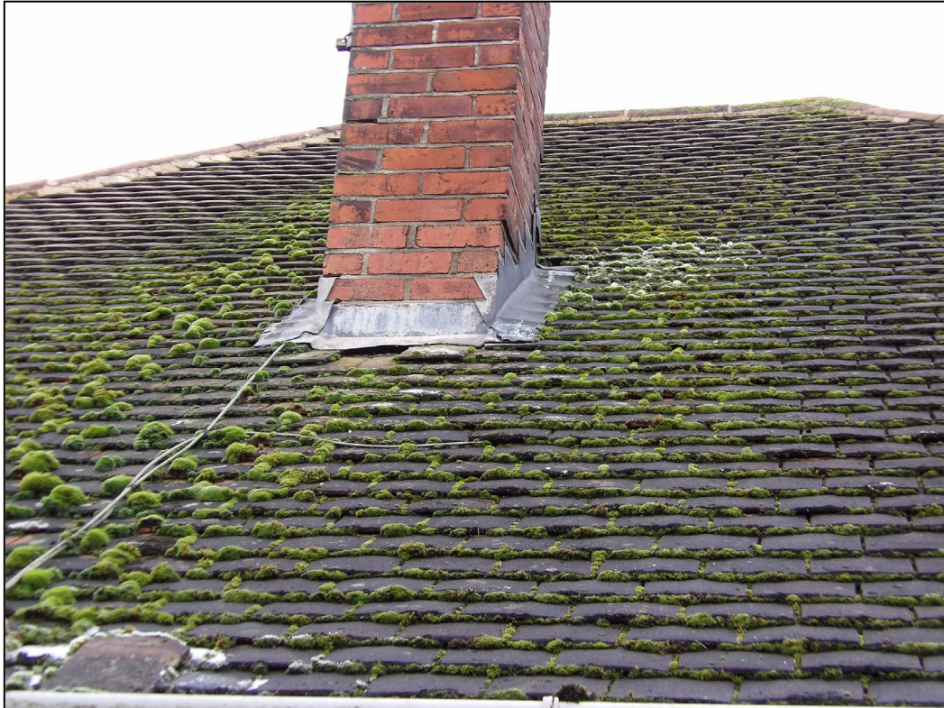
Figure 5. Example of slipped roof tile on east elevation. 108 Reading Road, Woodley. 10.01.25
