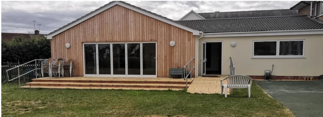
Fig 3. View of the rear (north) elevation of the site
