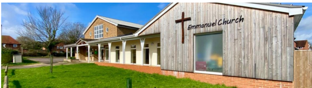
Fig 2. View of the front (south) elevation of Emmanuel Church Centre
