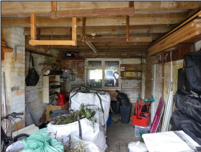
Figure 13. Internally view of garage and ceiling. 68 Arthur Road, Wokingham. 12.06.24
