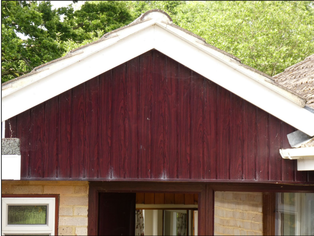
Figure 7. Example of close-fitting wooden cladding. 68 Arthur Road, Wokingham. 12.06.24
