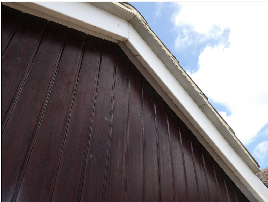
Figure 8. Example of soffits and fascias. 68 Arthur Road, Wokingham. 12.06.24
