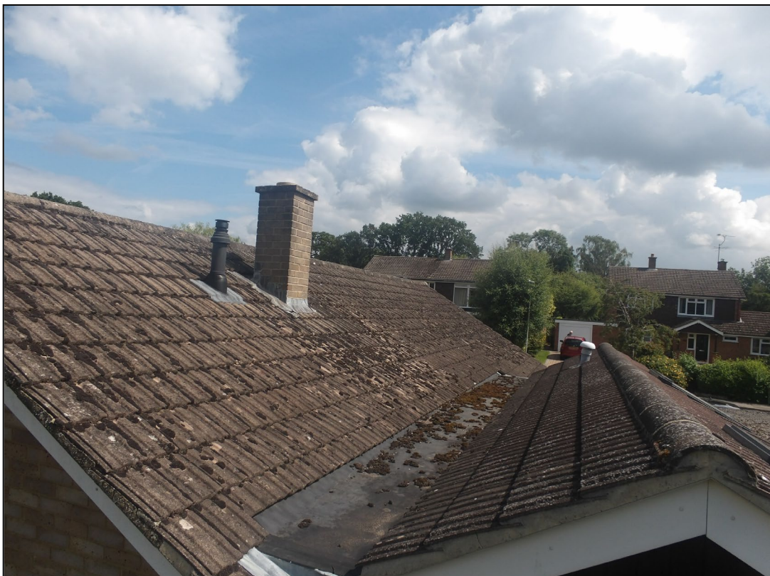
Figure 4. Tightly fitted roof tiles and lead flashing. 68 Arthur Road, Wokingham. 12.06.24
