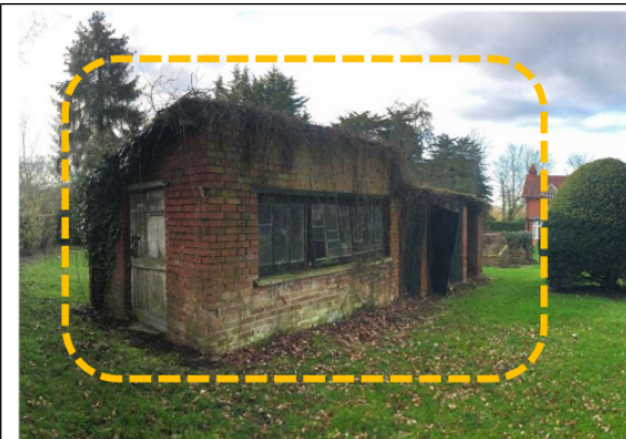
Figure 11 Outbuilding to be demolished
