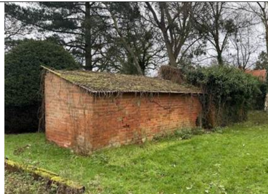
Figure 12 Outbuilding to be demolished
