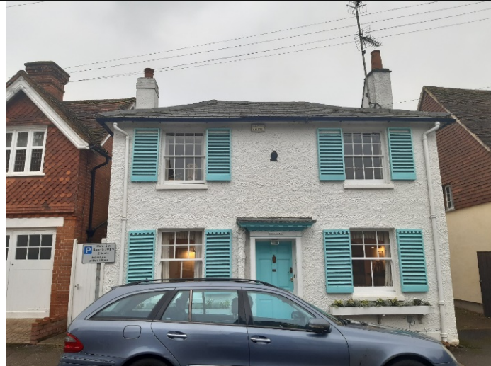
Figure 1 Front elevation of River Cottage
