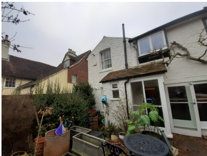
Figure 3 Rear elevation of River Cottage towards Gaunt House
