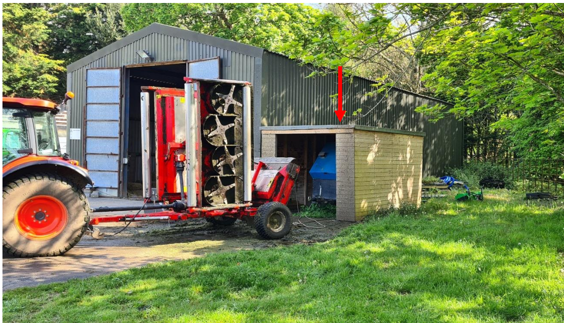
Fig. 1 – The open fronted storage shed (May 2024)
